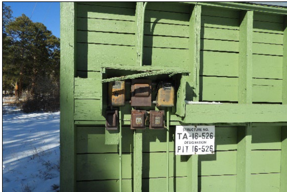
Figure 124. The top of the cover box is in need of repair.
