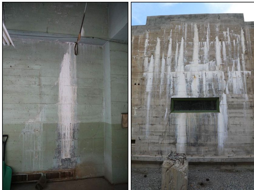
Figure 32. Examples of efflorescence on an interior wall and an exterior wall.
