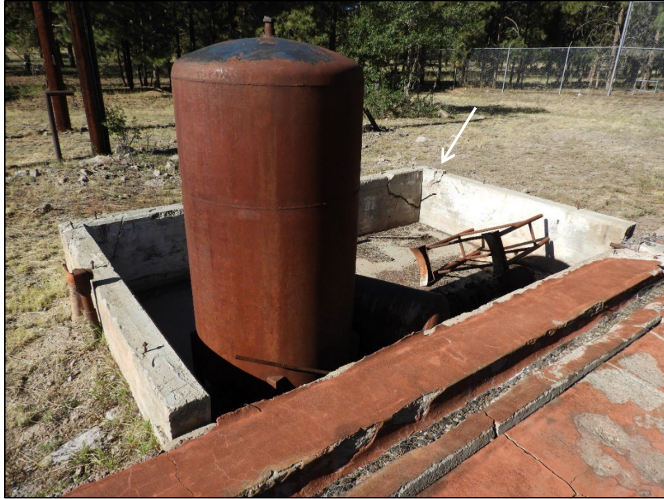
Figure 94. The corner separation is easily seen here in the southeast corner of the room.
