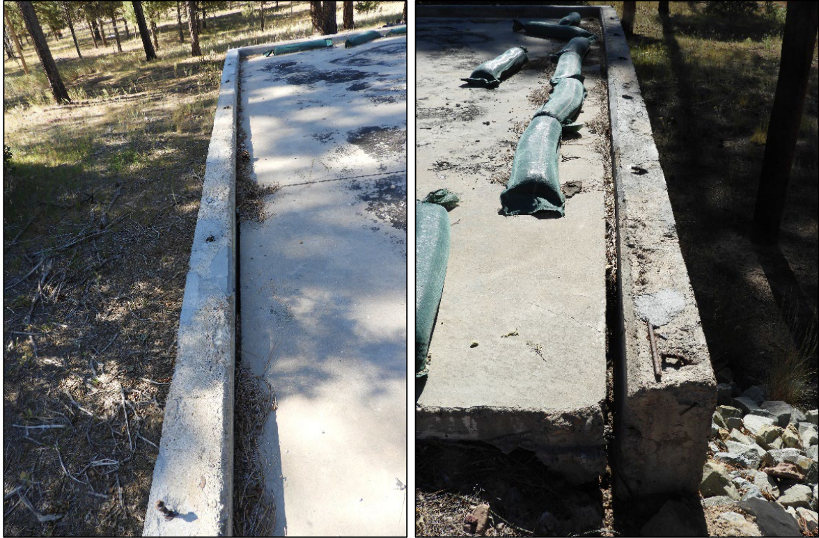
Figure 128. The separation extends most of the length of the wall.
