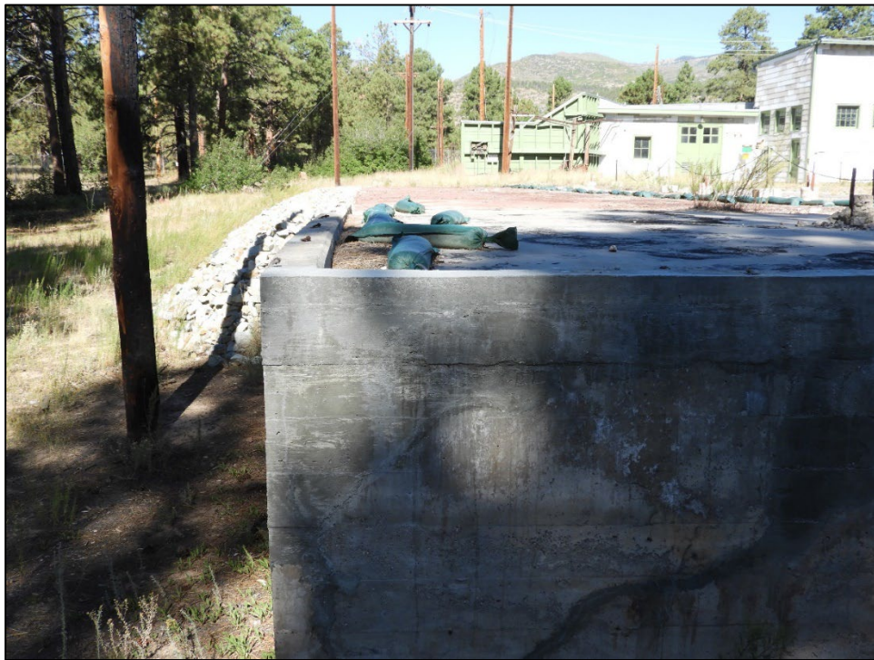
Figure 129. Photo shows the bulging stem wall along the south perimeter.
