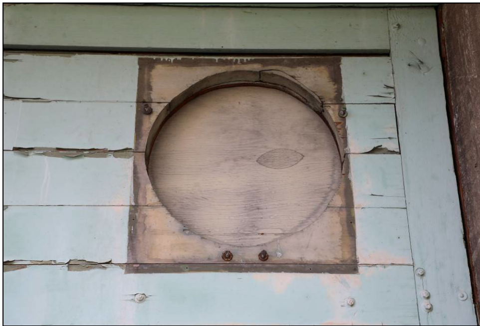
Figure 23. Exterior view of the duct hole and plywood cover.
