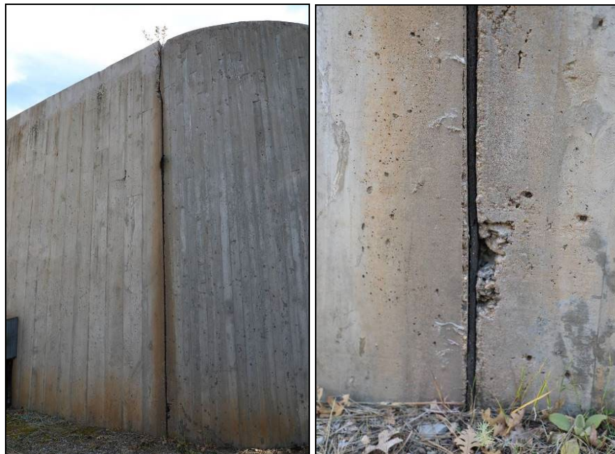
Figure 33. An overview shot of a typical vertical expansion joint to show height followed by a close up to show material color.
