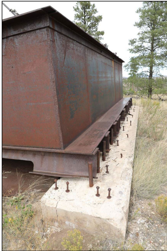
Figure 210. Oxidized metal that enters the interior of concrete often times has a detrimental effect on the preservation of the concrete.
