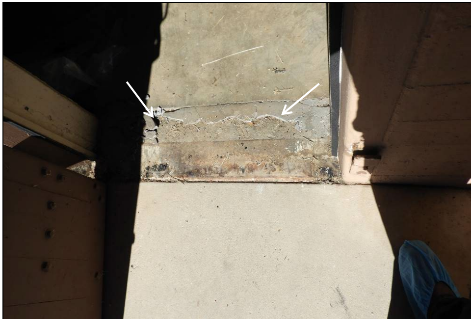
Figure 68. Patched concrete on the interior of the threshold is worn and presents a trip hazard.
