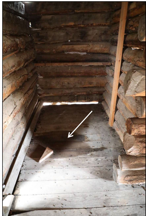
Figure 181. Arrow points to evidence of an active roof leak.
