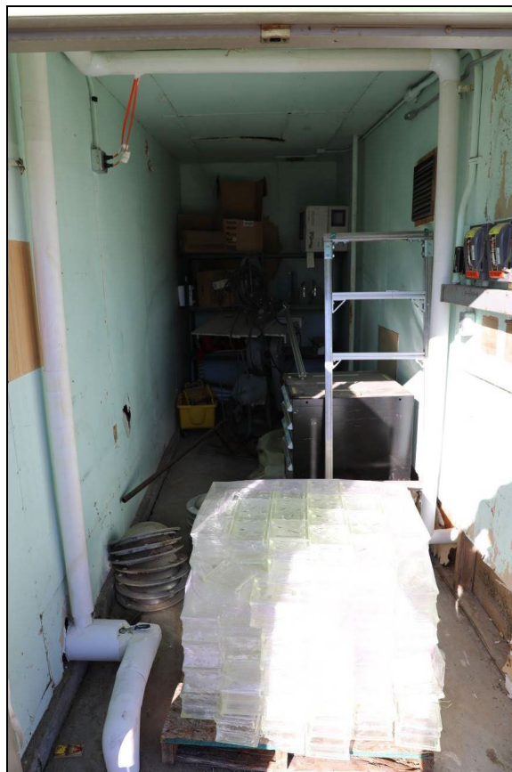
Figure 84. The newly insulated plumbing can be seen in white in the foreground of the photograph. Still-to-be-repaired water damage can be in the bottom right hand corner.
