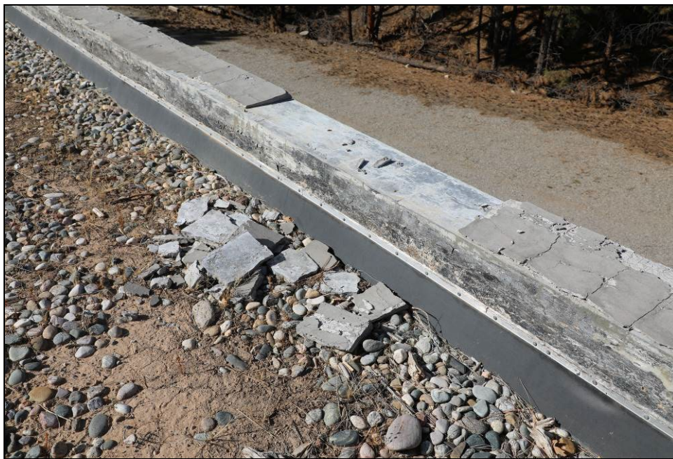
Figure 34. An example of the failing parapet cap.
