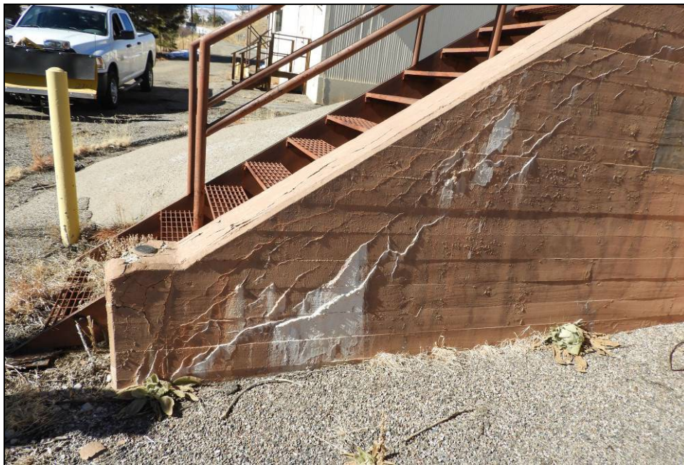
Figure 67. Efflorescence is present on the exterior of the east wing wall.
