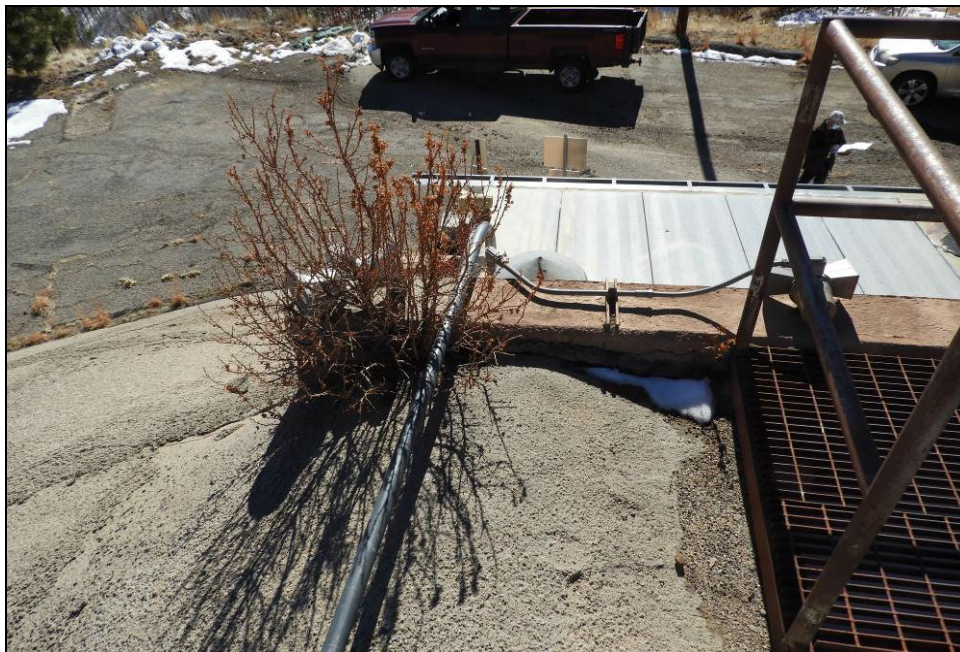
Figure 73. The shrub is growing up against the parapet and causing damage to the original architecture.
