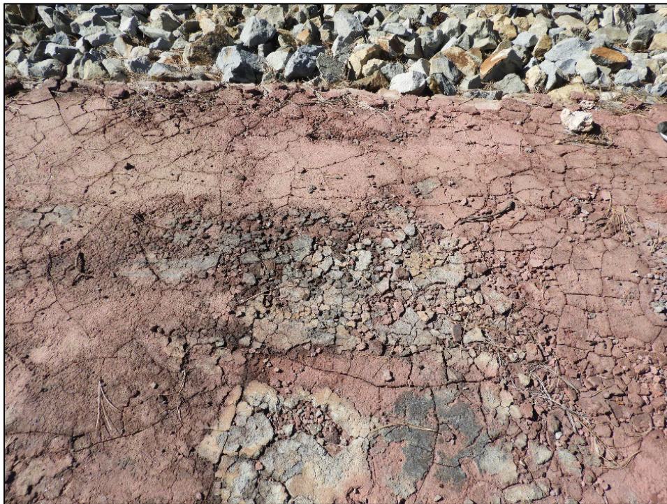
Figure 132. Cracking and general deterioration of the Hubbelite are severe.
