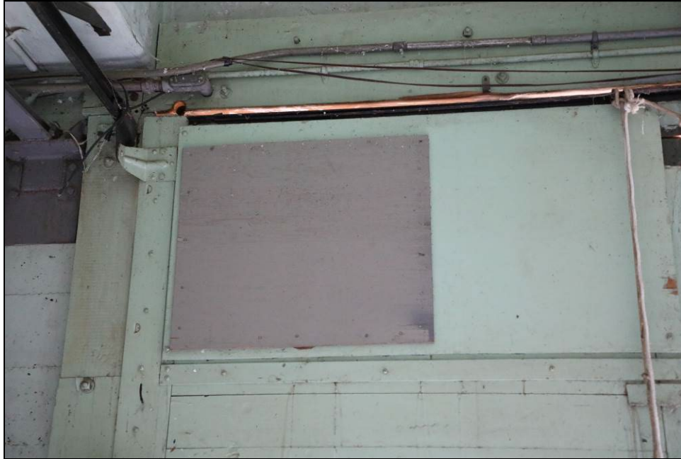
Figure 22. Interior view of the plywood piece covering the round ducting hole.
