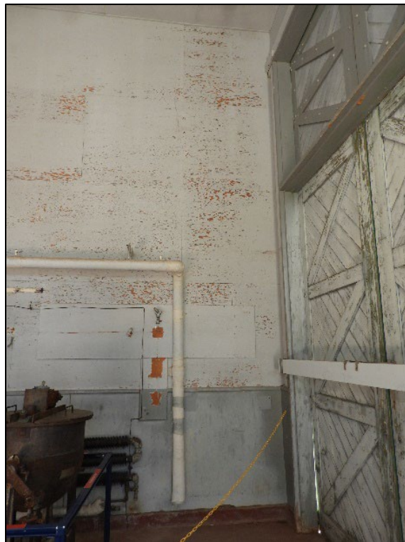
Figure 110. The underlay of the plywood sheathing is becoming exposed as the paint flakes away from the surface.
