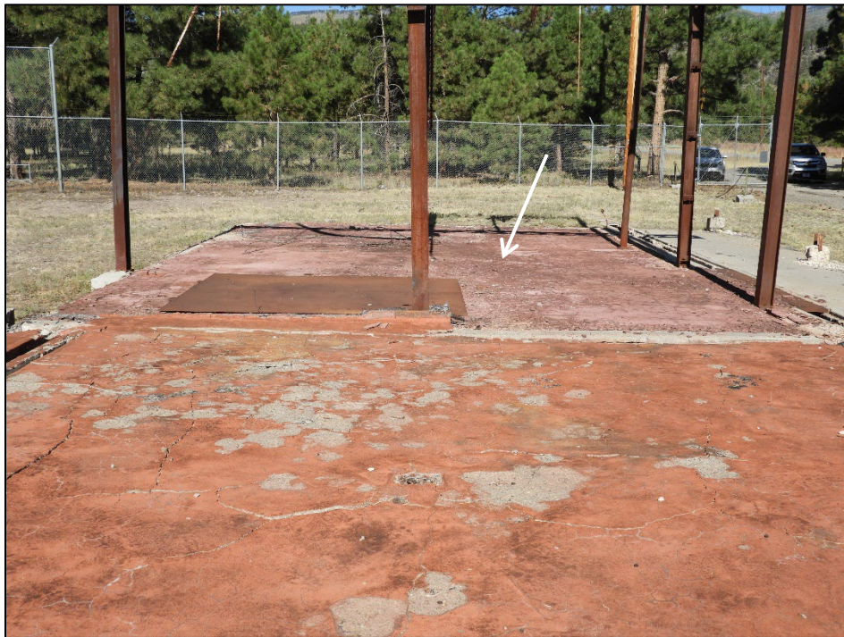
Figure 91. The Hubbelite pad is farther pad in the photograph. Chipping and breakage is severe and likely releases low levels of asbestos into the nearby environment.
