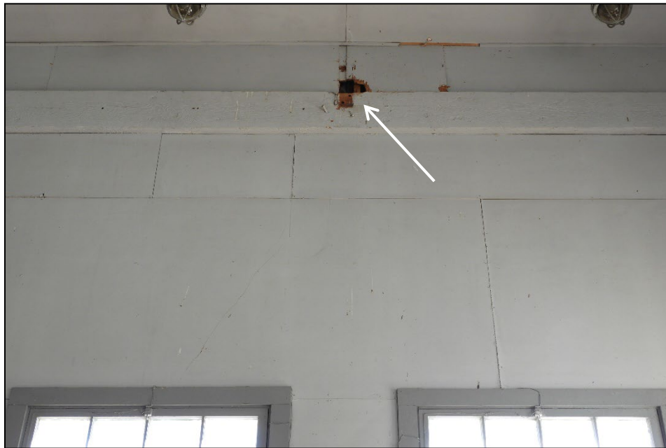
Figure 108. The small hole allows access to the interior of the walls.
