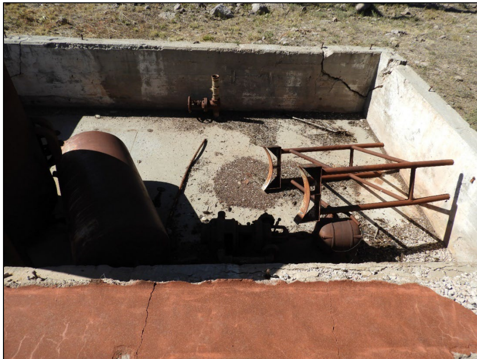
Figure 92. Debris has collected on the surface of the floor; trapping moisture and presenting an untidy appearance.
