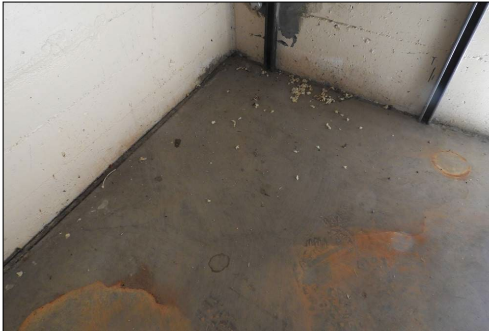
Figure 69. Rodent debris scattered under vent and utility hole openings to the left of the entrance door.
