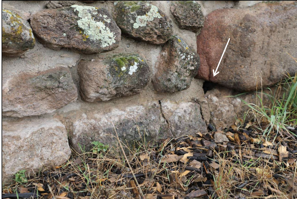
Figure 191. Minor voids can also be found on the exterior of the chimney.
