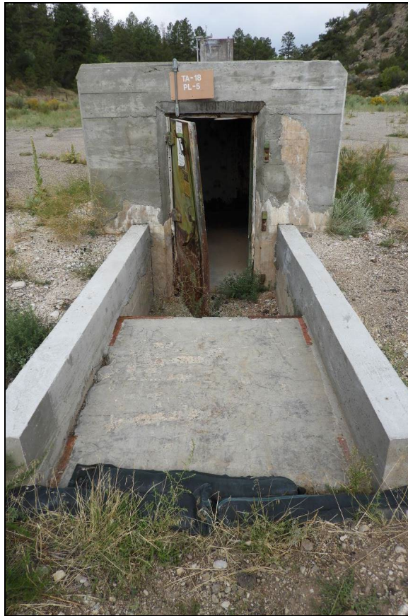
Figure 177. The block is in-place of stairs and should be removed.
