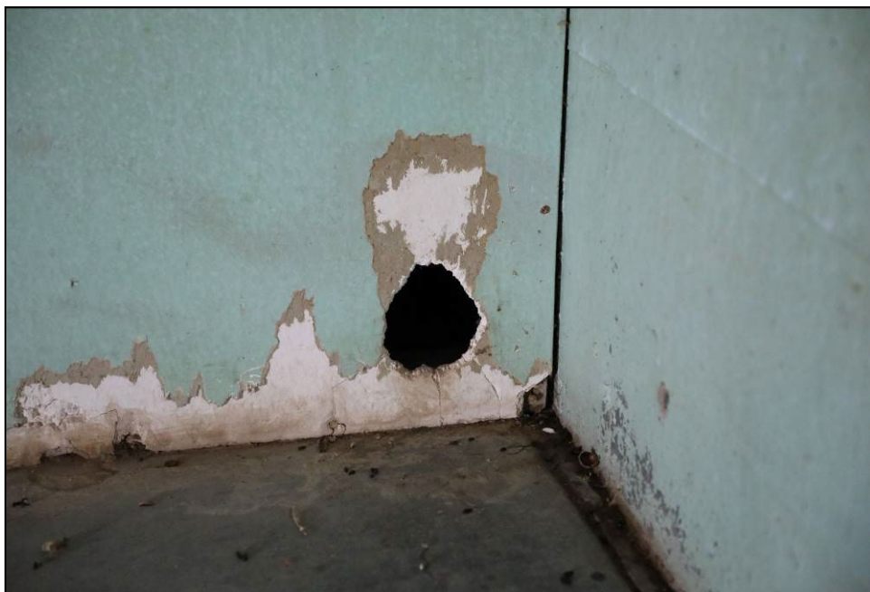
Figure 9. Holes like this one allow rodents an nice place to nest and reproduce.
