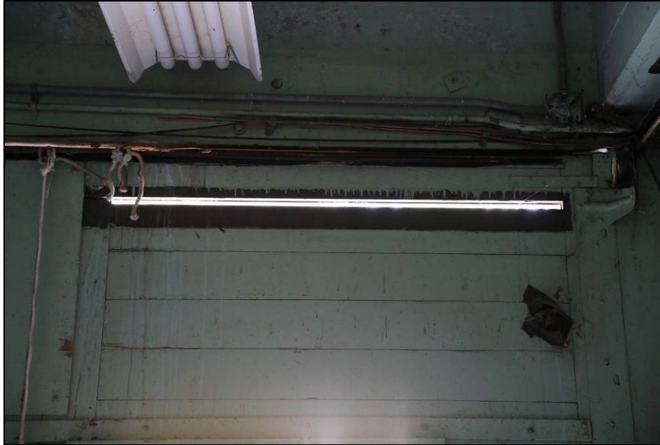
Figure 18. Daylight can be seen through the separation above the bay door.
