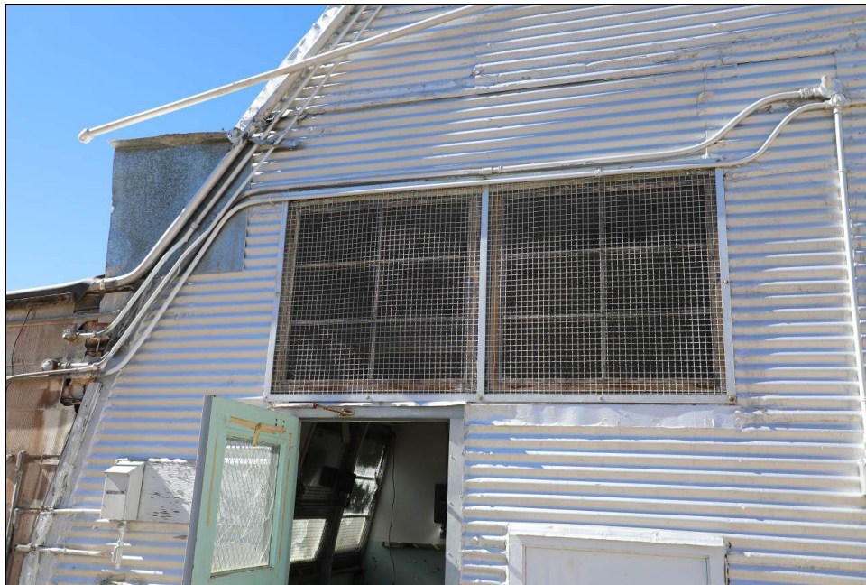
Figure 203. The window opening above consists of only screen material.
