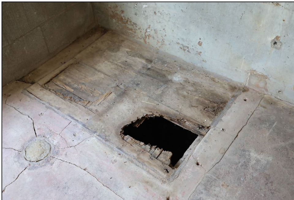
Figure 43. The plywood cover that once successfully covered the utility pit no longer functions properly.
