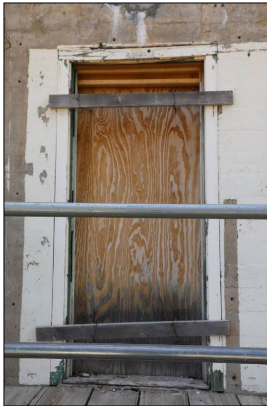
Figure 47. Exterior photograph of the door opening needing a reconstructed door.
