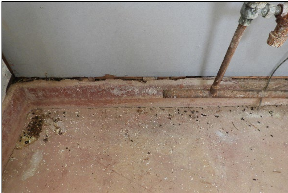
Figure 109. Photo shows cracking of the baseboard that allows rodent access to the interior of the wall.
