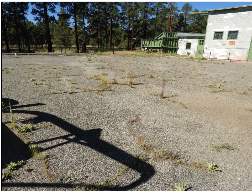
Figure 137. Water drains to the original concrete pad in front of 16-0517 and threatens the preservation of the doors and the interior of the building.
