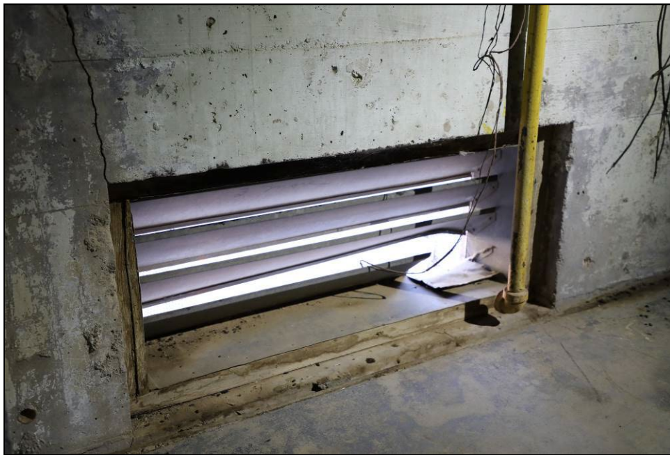
Figure 15. The broken louver is unsightly and the worn screen cover needs replacement.
