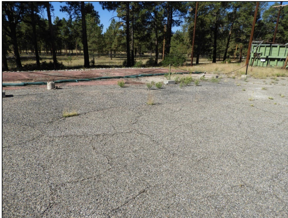
Figure 136. Drainage to the Hubbelite pad of 16-0519 and 16-0520 present significant preservation challenges.
