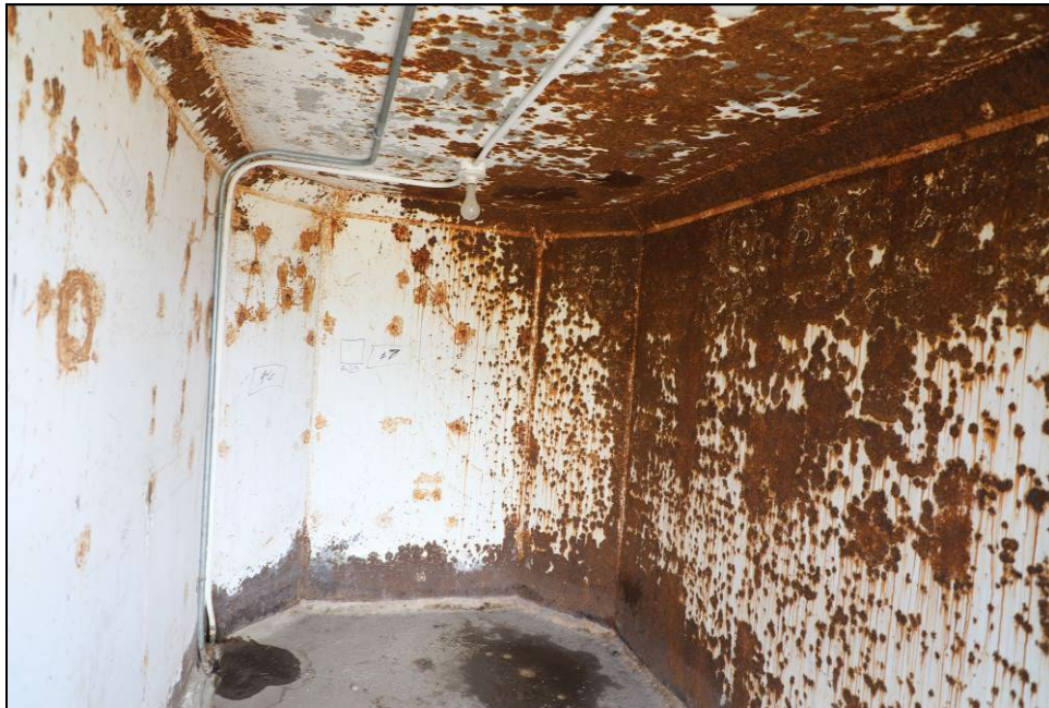
Figure 176. Rust is prevalent throughout the interior.
