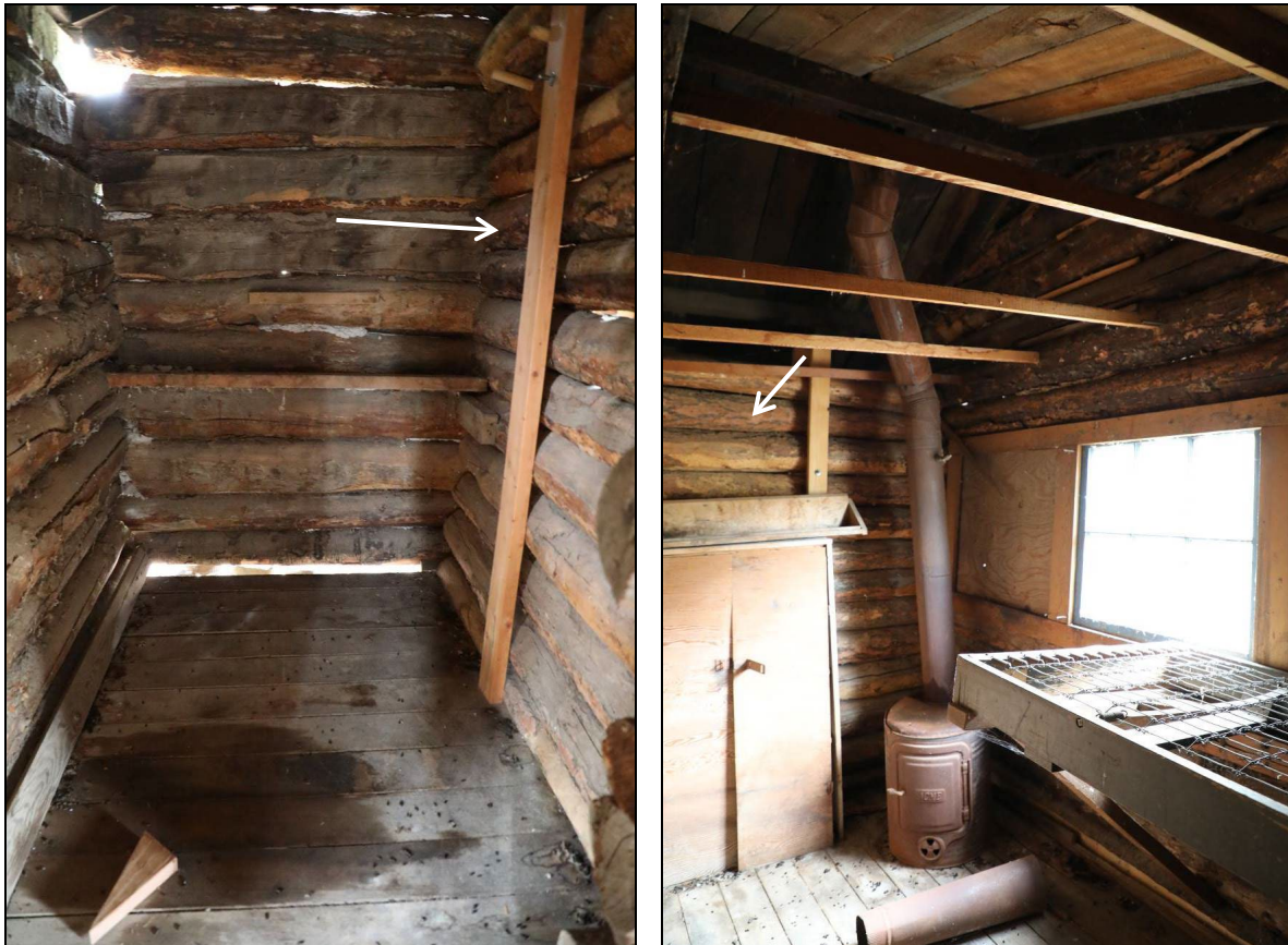
Figure 185. Arrows point out the interior log wall.
