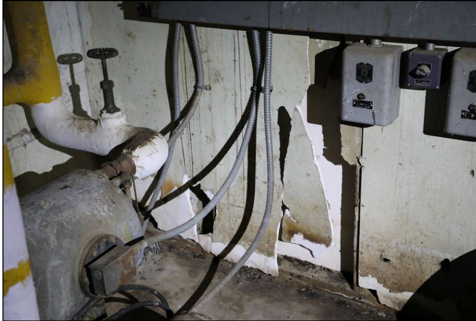
Figure 12. Whole sections of interior siding will need replacement.
