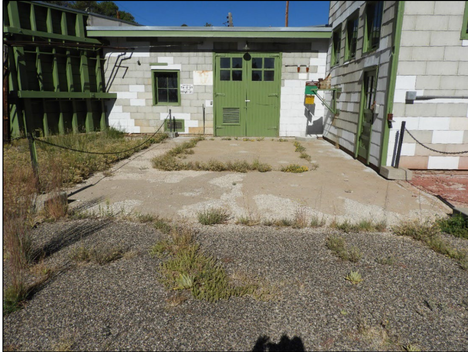
Figure 137. Water drains to the original concrete pad in front of 16-0517 and threatens the preservation of the doors and the interior of the building.
