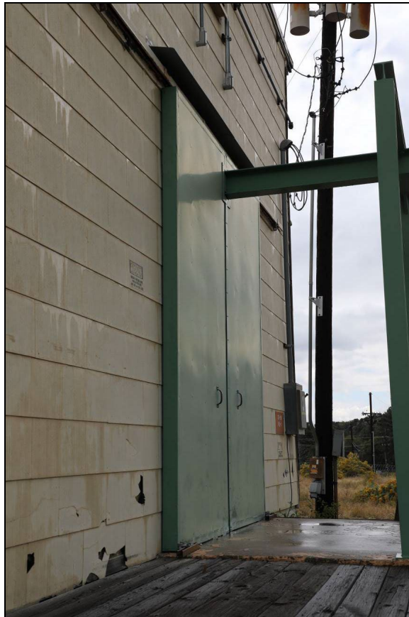
Figure 162. The large bay doors after a rain. Water was noticed to be leaking into the building from the top of the doors.
