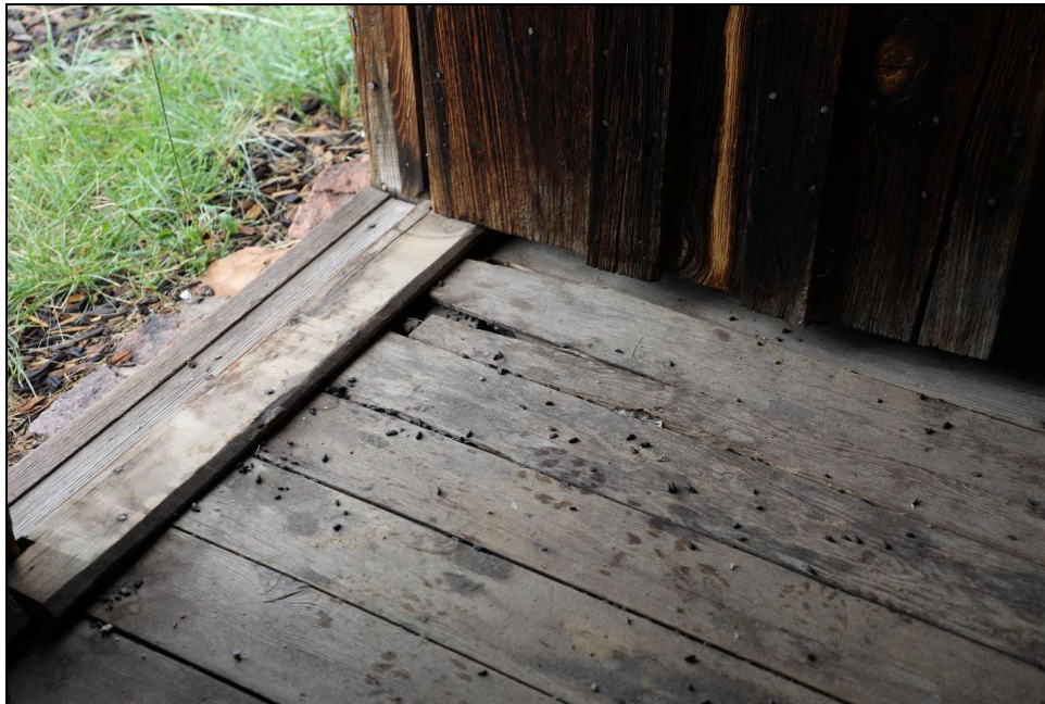
Figure 194. Photograph illustrates a typical section of flooring in need of repair.
