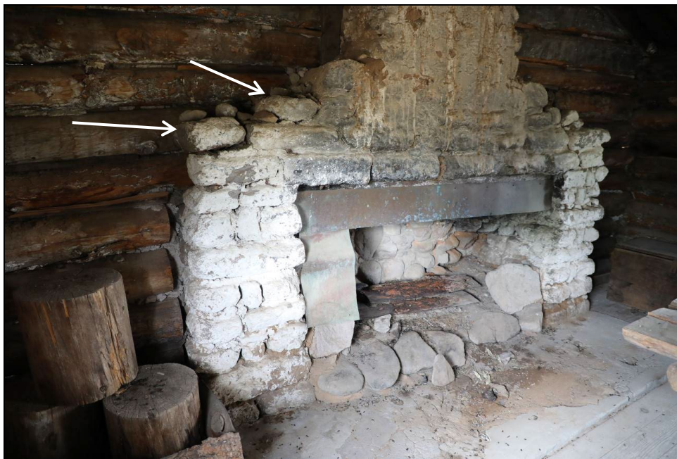
Figure 190. Arrows point to the loose stone visible in the photograph.
