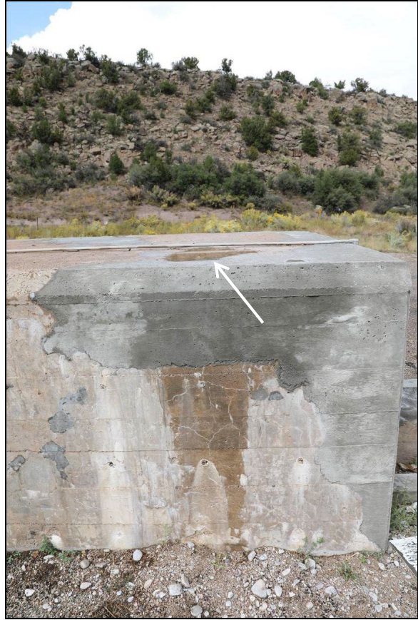
Figure 175. Photographs show active leaks and standing water on the roof.
