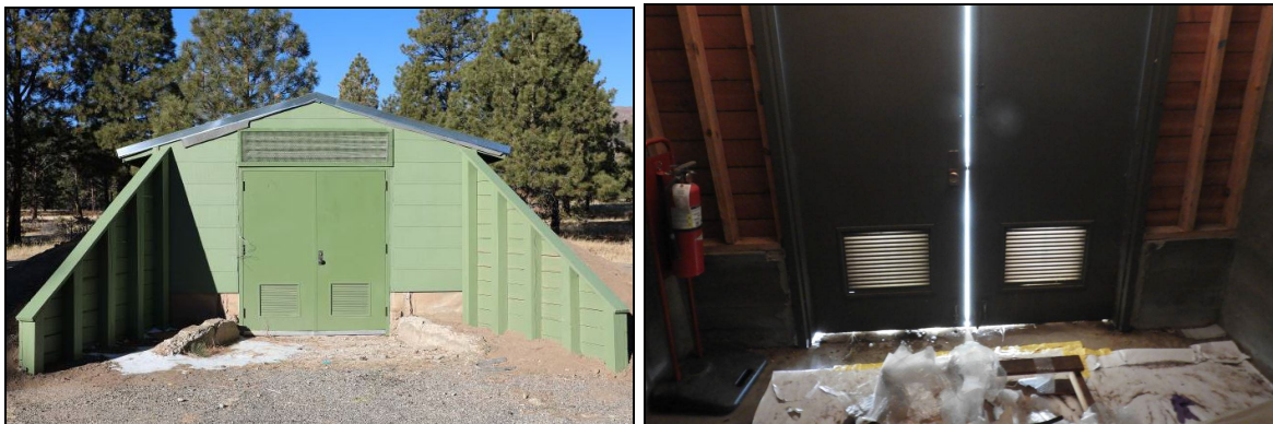
Figure 150. The non-original doors do not provide a proper fit to keep out pests.
