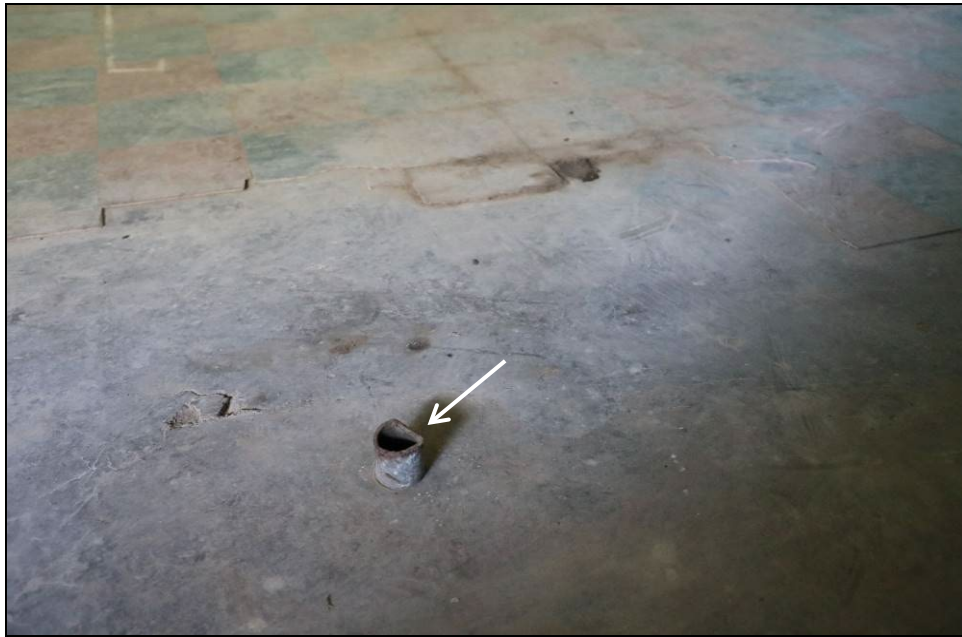
Figure 31. An old utility conduit rises up out of the floor and presents a substantial tripping hazard.
