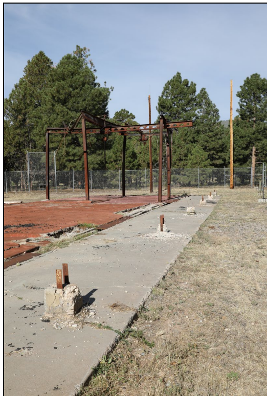
Figure 88. The line of concrete bases used to support bracing that held up an overhang.
