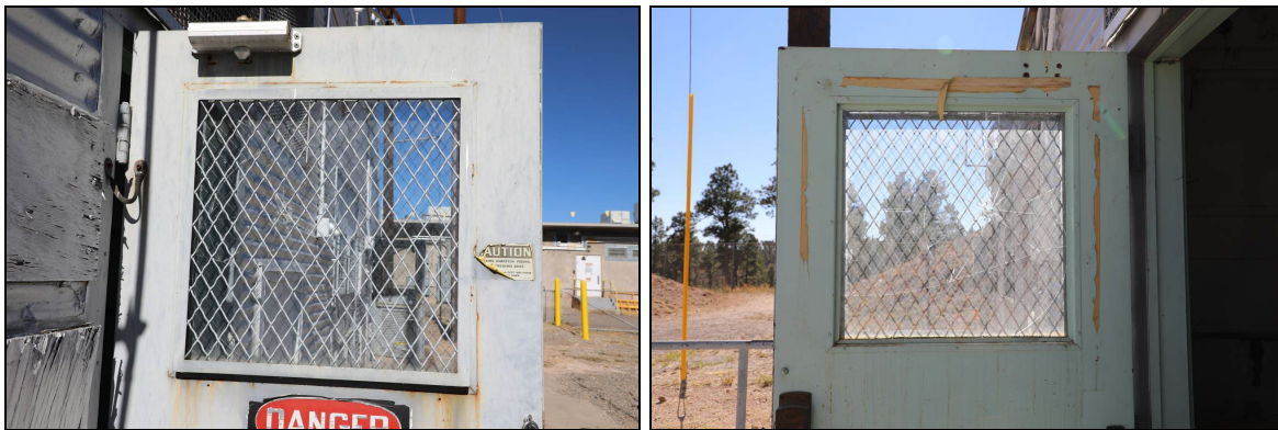
Figure 201. Photograph showing the shattered glass in the east elevation door.
