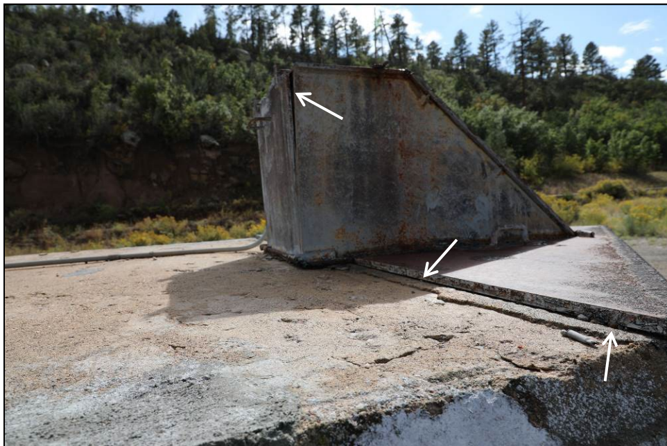
Figure 174. Photograph shows the areas where leaks have been identified.
