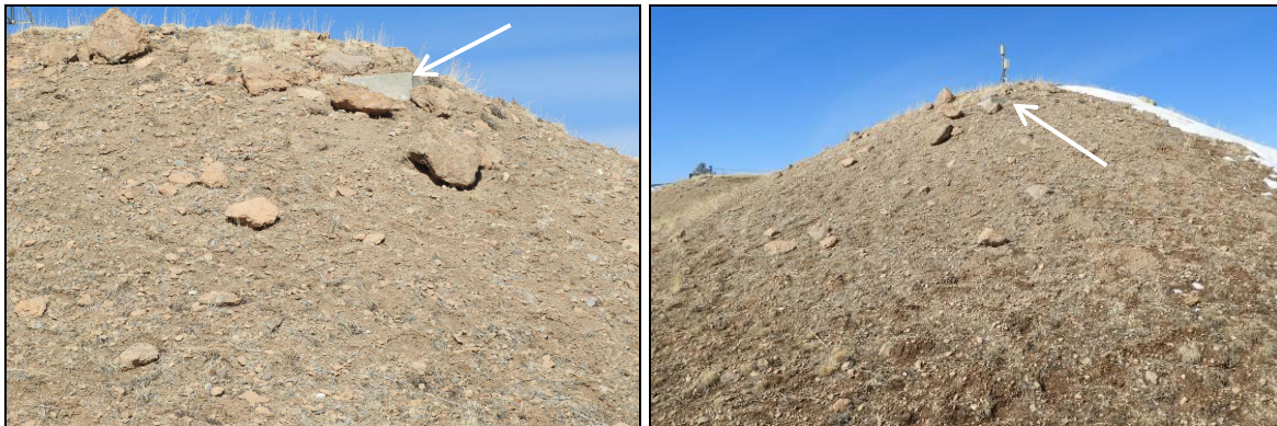
Figure 55. Arrows point to the exposed concrete roof corners on the southeast and northeast corners.
