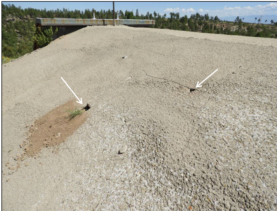
Figure 59. Active burrowing is evident in this recent photo.
