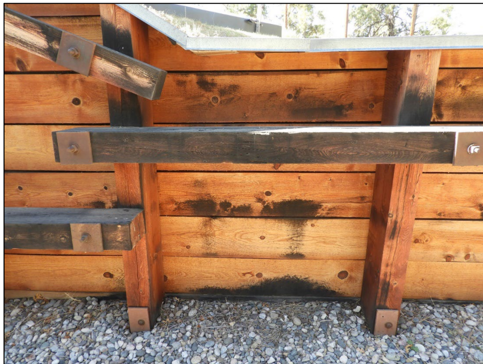
Figure 141. Close-up of a section of the fence to highlight extent of biological growth.
