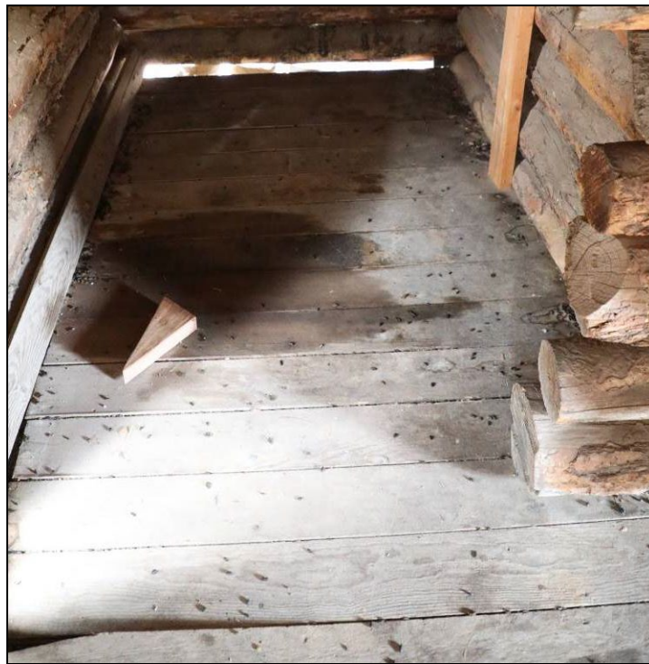
Figure 193. Photograph shows rodent droppings scattered across the floor.
