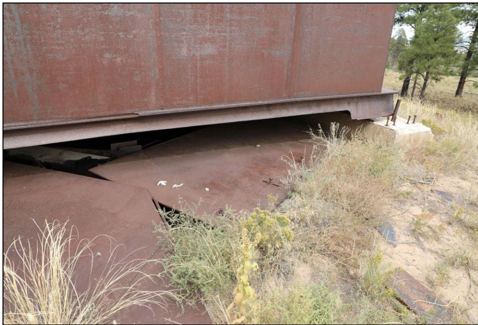
Figure 213. The side opening allow wildlife access to the bottom of the pit. This will be harder to close off compared with the top hole.
