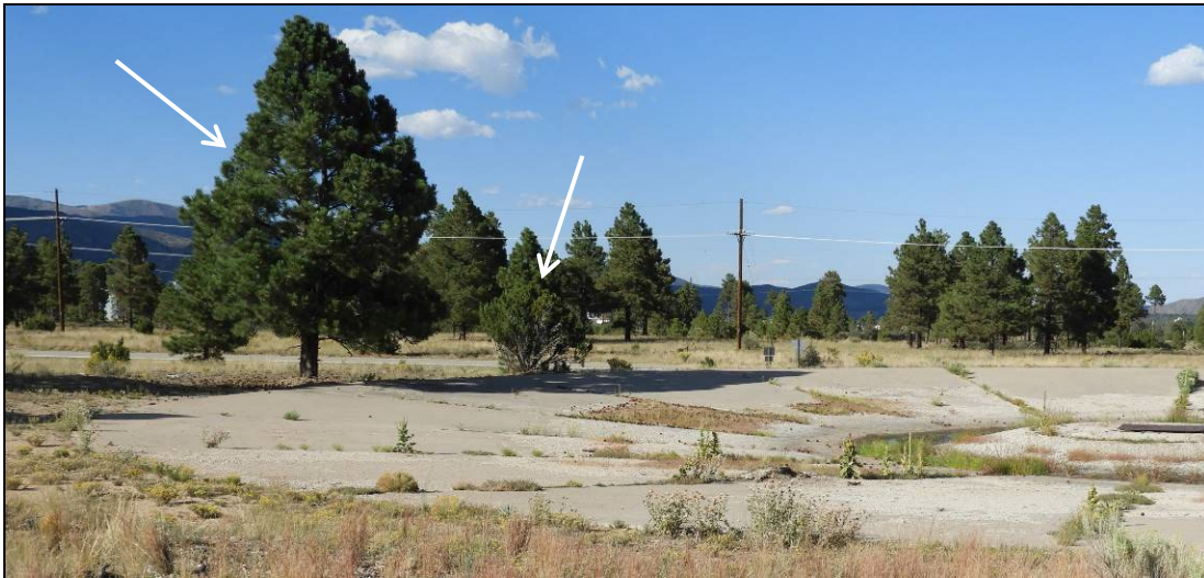
Figure 3. The two trees create uplift on the nearby concrete slab and deposit duff on top of the Concrete Bowl.
