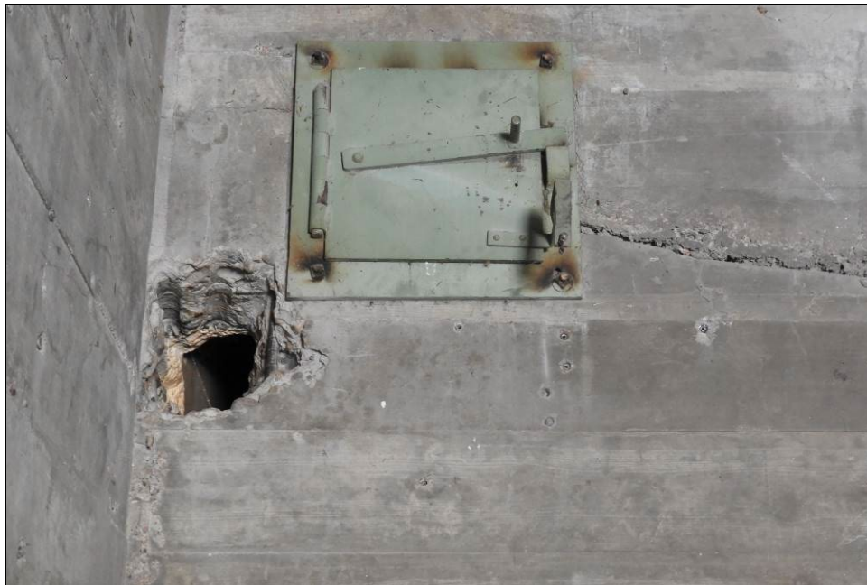
Figure 60. Utility hole with conduit no longer occupying it.
