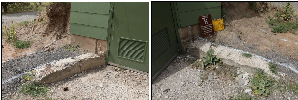
Figure 155. The original wing wall foundations are in poor condition, but still exhibit the original post holes for the vertical support beams.
