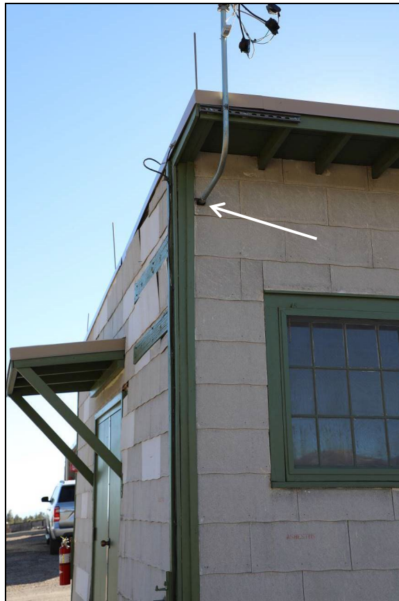
Figure 83. Conduit and related hole can be seen exiting the building in the upper corner of the north elevation.
