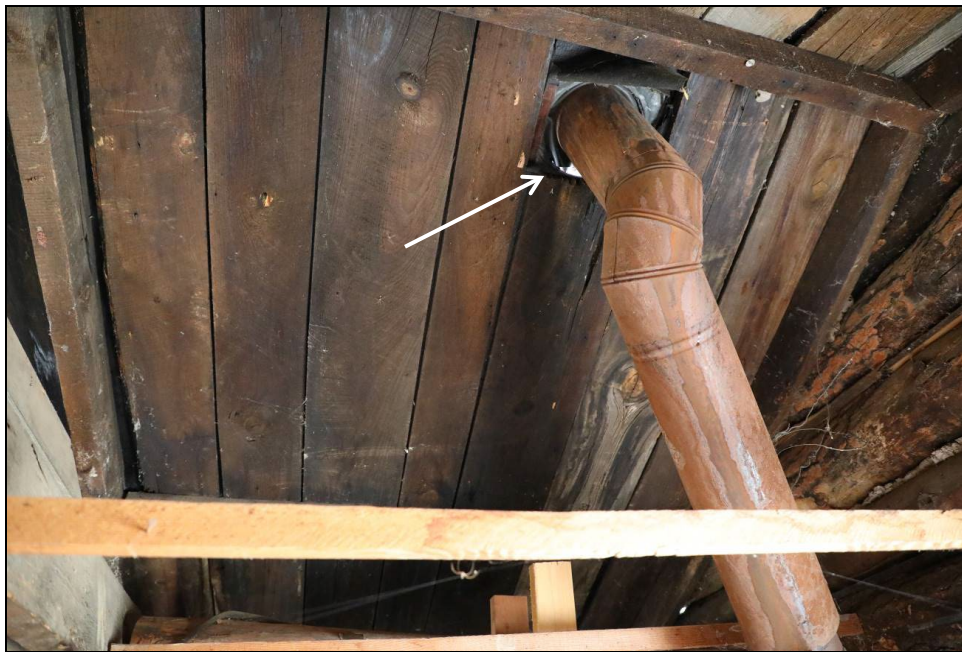
Figure 182. Arrow points to daylight as seen around the stovepipe penetration from the inside of the cabin.
