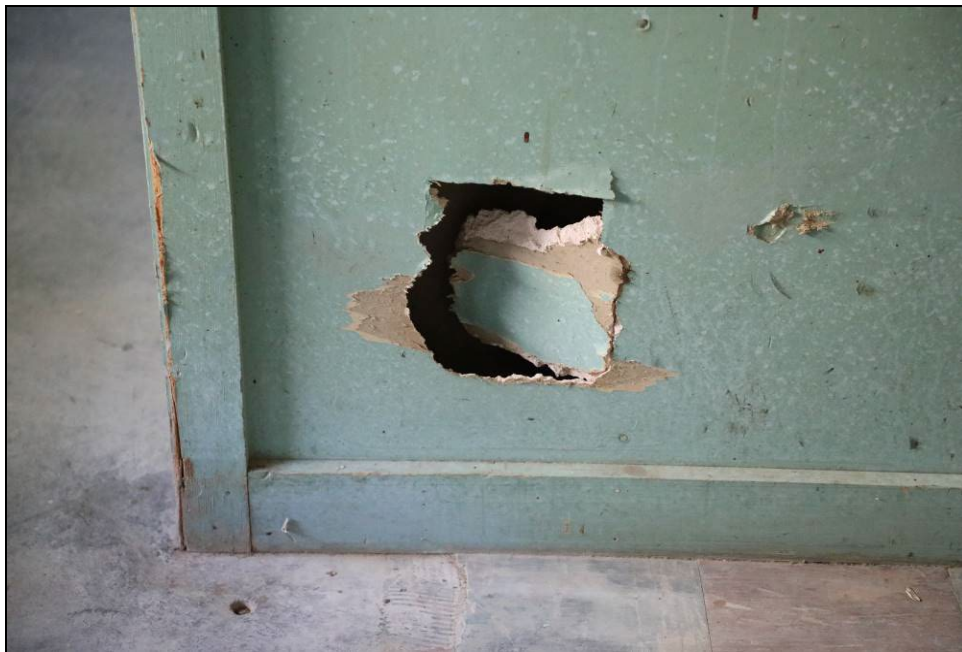
Figure 11. This example is fairly typical of the types of holes throughout the building.
