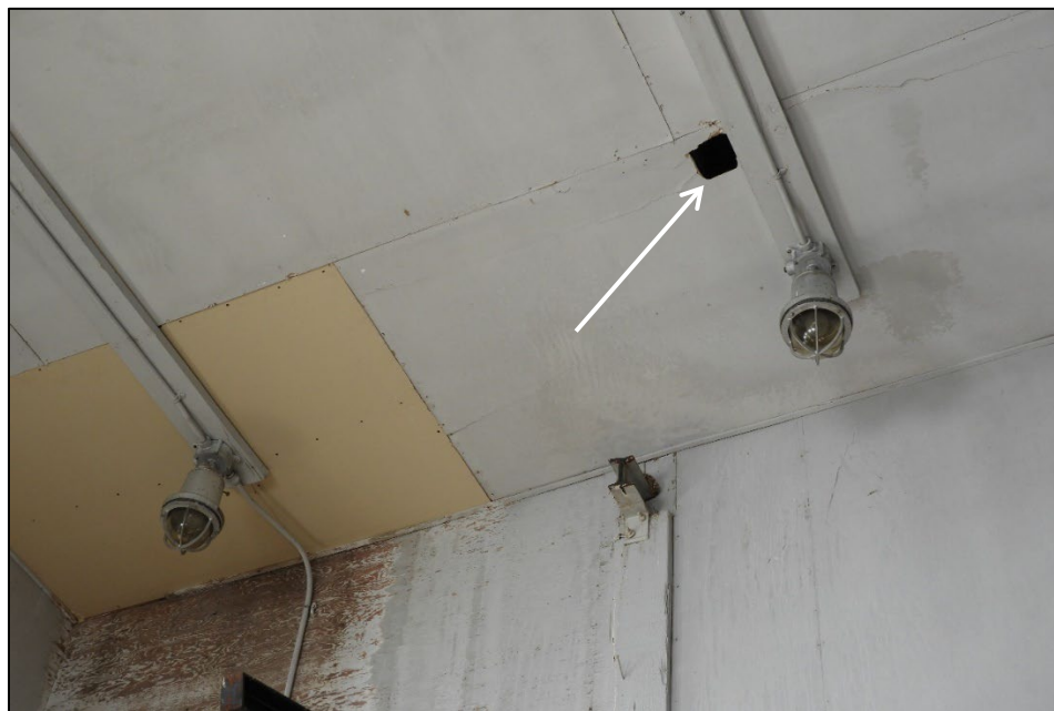
Figure 103. The 5" x 5" hole in the ceiling requires a patch - a difficult task, but achievable.
