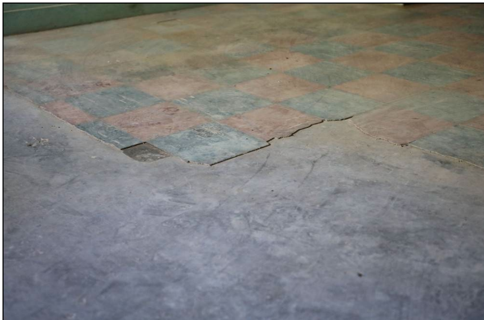
Figure 30. The 8" x 8" asbestos tiles are cracking and breaking apart at the edges.
