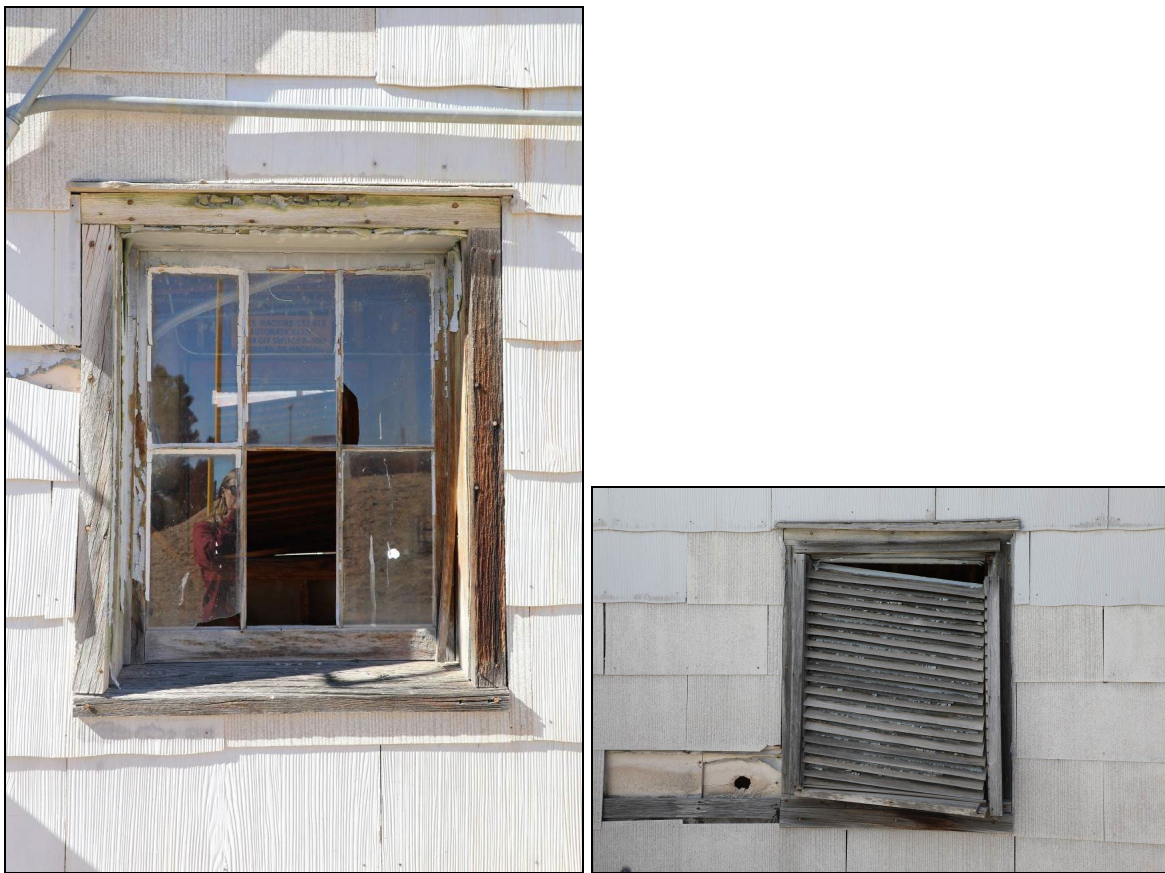
Figure 207. The east elevation window opening (left) and the west elevation opening (right) will require extensive work.
