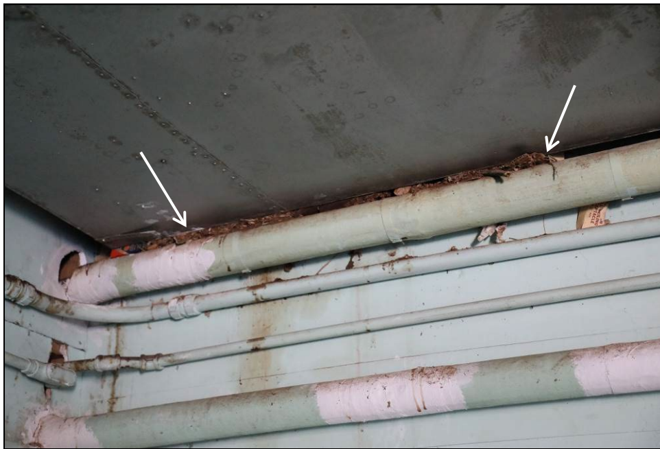
Figure 13. A large pack rat nest is visible on top of utility line that has a larger-than-needed penetration hole through the wall.
