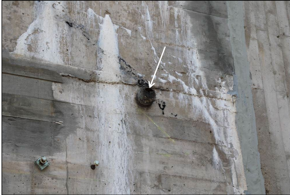
Figure 16. The screen covering this wall penetration is cracked and aged; allowing access for pests to the inside.
