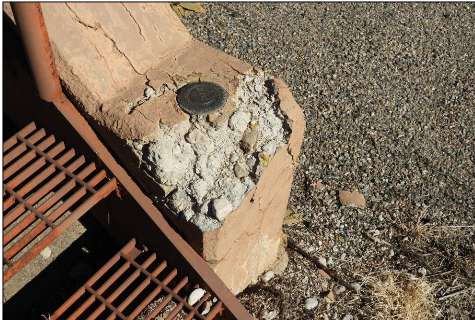
Figure 65. Major concrete deterioration is occurring near the benchmark on the west wing wall.
