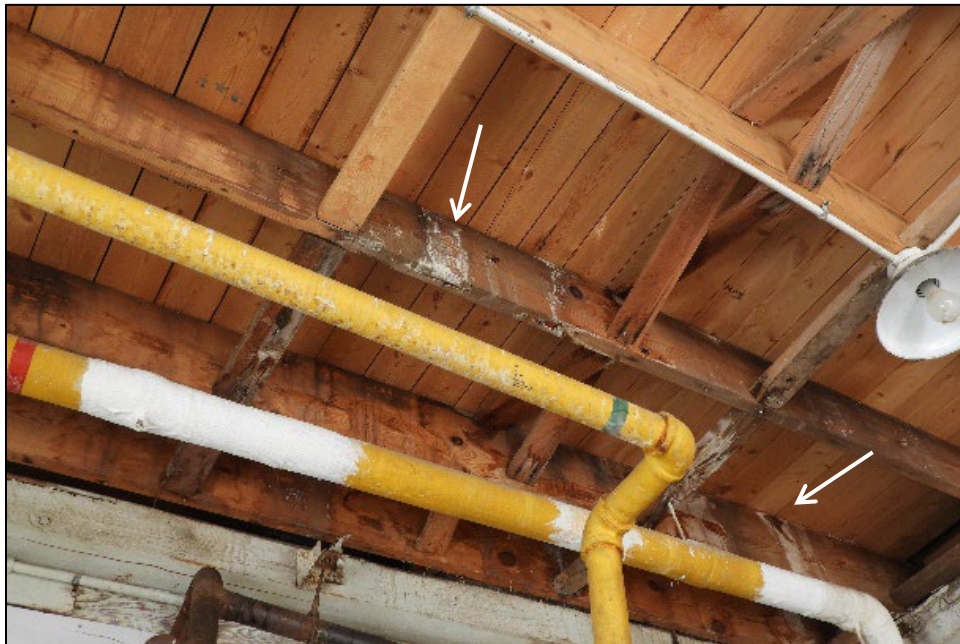
Figure 115. Evidence of recent leaks are evident on the ceiling joists and roof decking.
