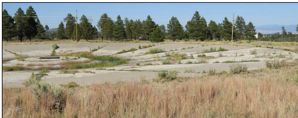
Figure 2. The majority of the vegetation growth occurs in the expansion joints seen here as green lines radiating out from the center.
