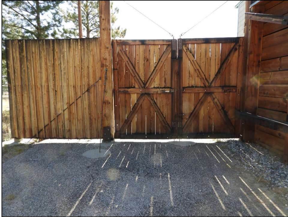
Figure 140. Exterior view of the gates and no-peek fence. Blackened areas on the wood represent biological growth.
