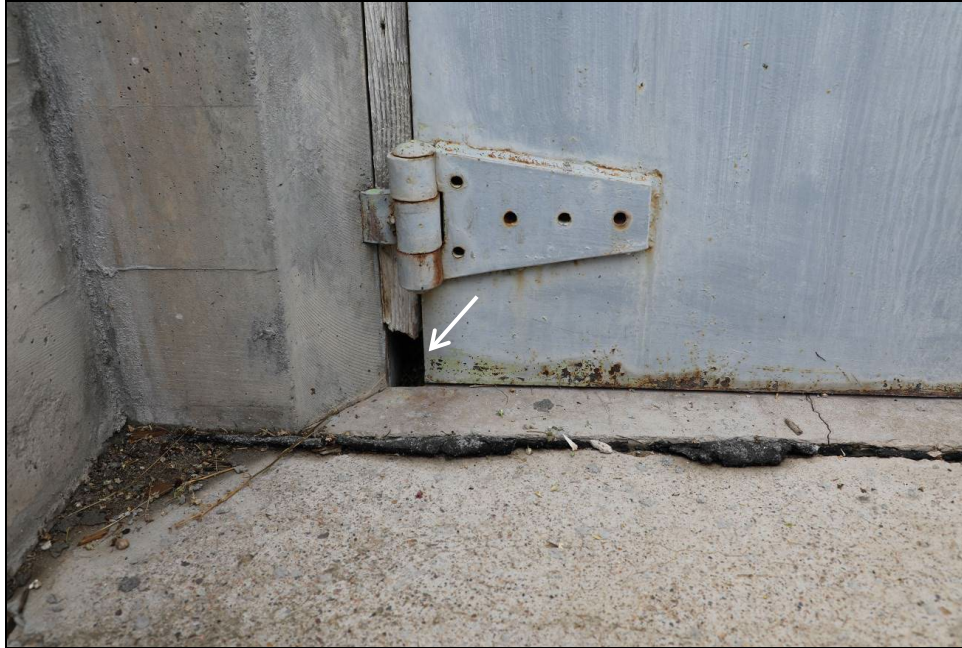
Figure 169. Close-up view of the missing piece of the frame.
