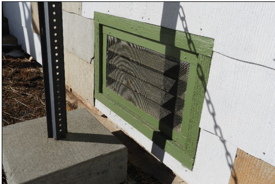
Figure 118. Screen over the louvered vent has aged and needs replaced.
