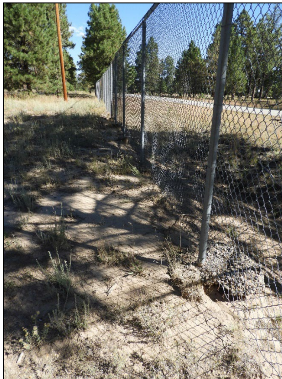
Figure 143. Erosion at the base of the fence may cause the fence to topple in the future.
