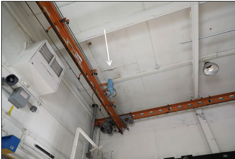
Figure 163. Damage from a previous roof leak in the southwest corner of the building.
