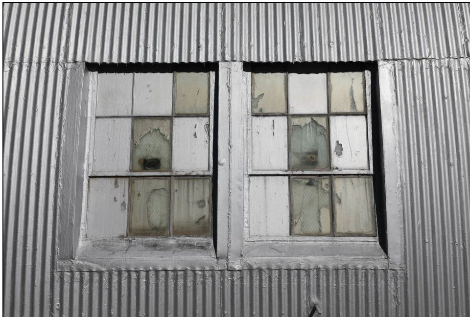
Figure 202. An example of metal windows requiring preservation work.
