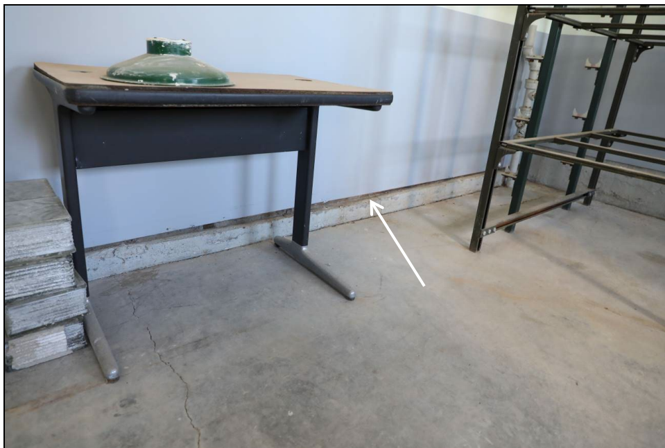
Figure 82. A long-running void can be seen just above the concrete base and the interior siding.
