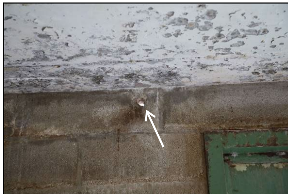
Figure 42. Example of a utility hole with the conduit removed.
