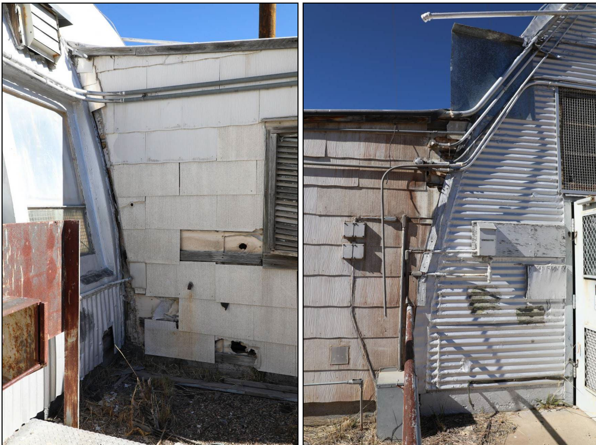
Figure 204. The utility annex has separated from the main building.
