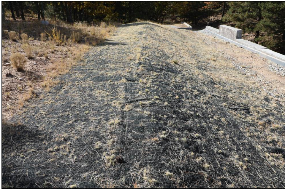
Figure 35. View of installed matting and degree of vegetation growth since 2012.
