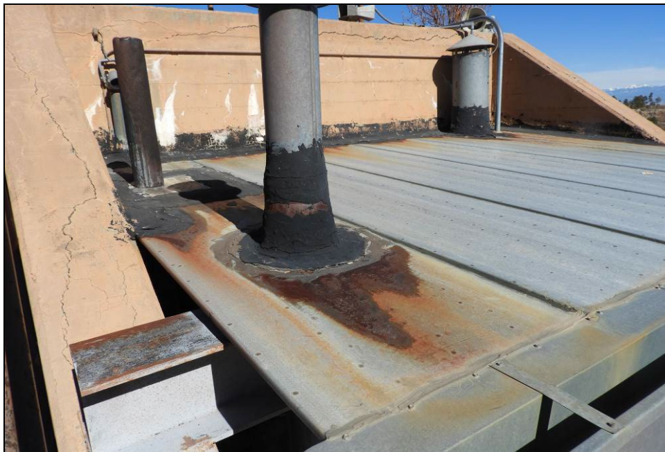
Figure 71. The age of the sealant around the points of penetration can be seen in this photo.
