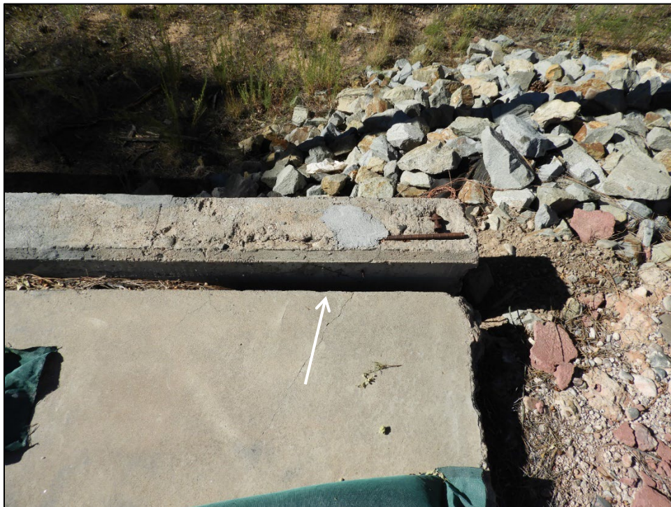
Figure 127. The photo shows the slab separation from the stem wall from above.
