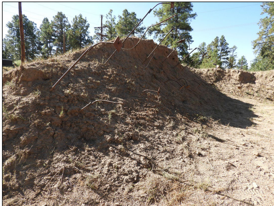
Figure 100. Profile shot of the east interior of the berm shows the extent of slope and lack of erosion controlling vegetation.
