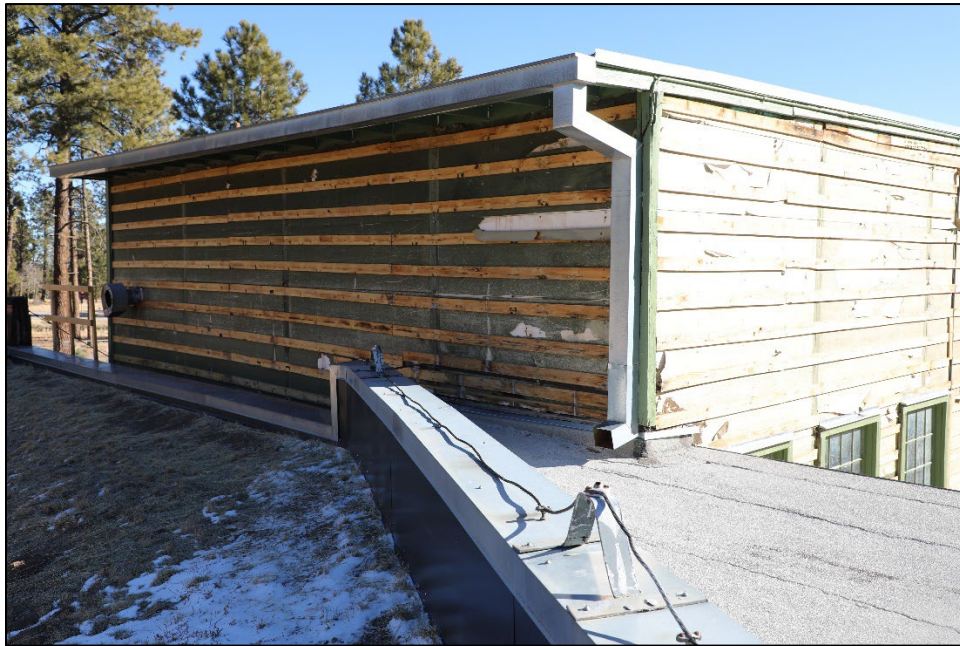
Figure 102. Photo shows the current drainage system from 16-0516 on to the roof of 16-0517.
