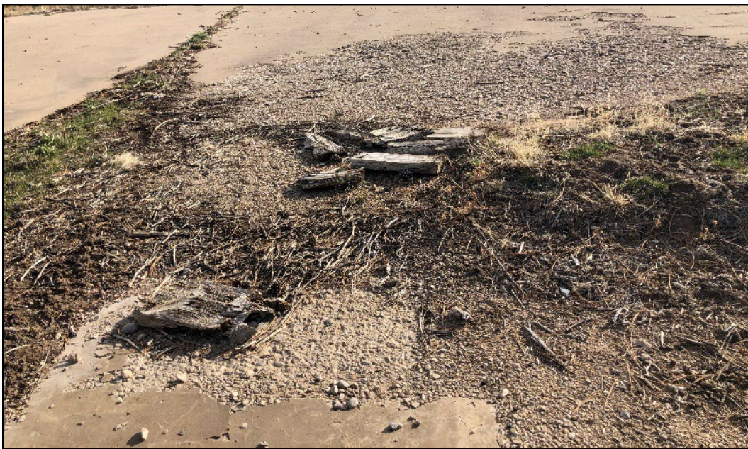
Figure 4. Extreme friability is exhibited in the photograph - a typical occurrence on the surface of the Concrete Bowl.
