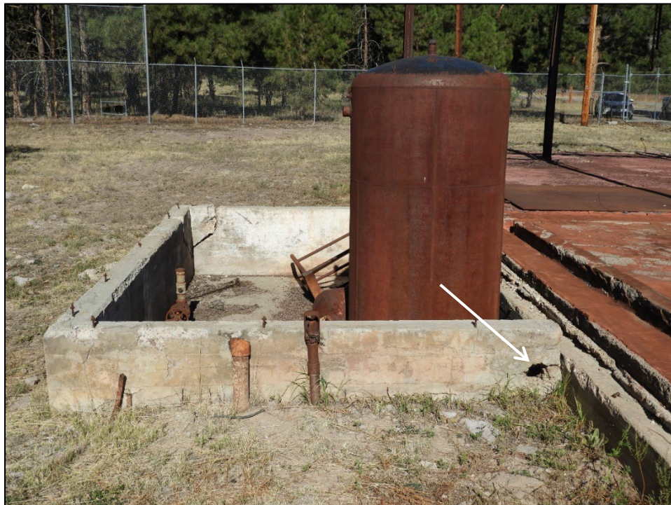
Figure 95. A large utility hole was chipped out of the northeast corner of the room.
