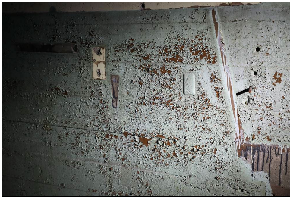
Figure 26. Example of peeling interior paint.
