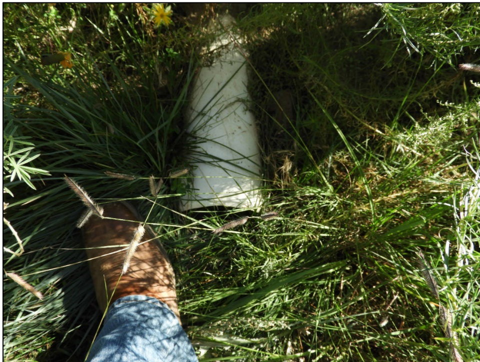
Figure 122. Drainage pipe needs a hardware cloth cover that can be easily removed if clogging occurs.
