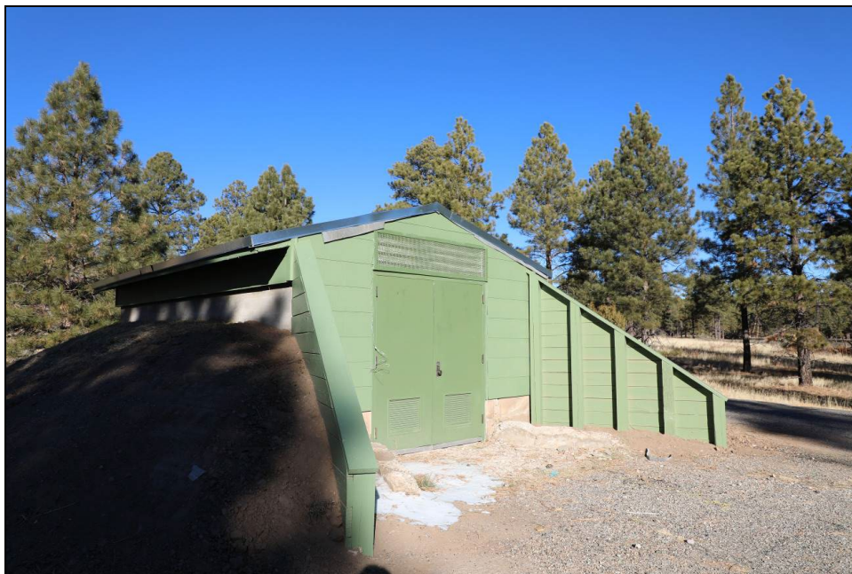
Figure 153. Photo shows that moisture accumulates near the entrance and requires a way to drain away from the building.
