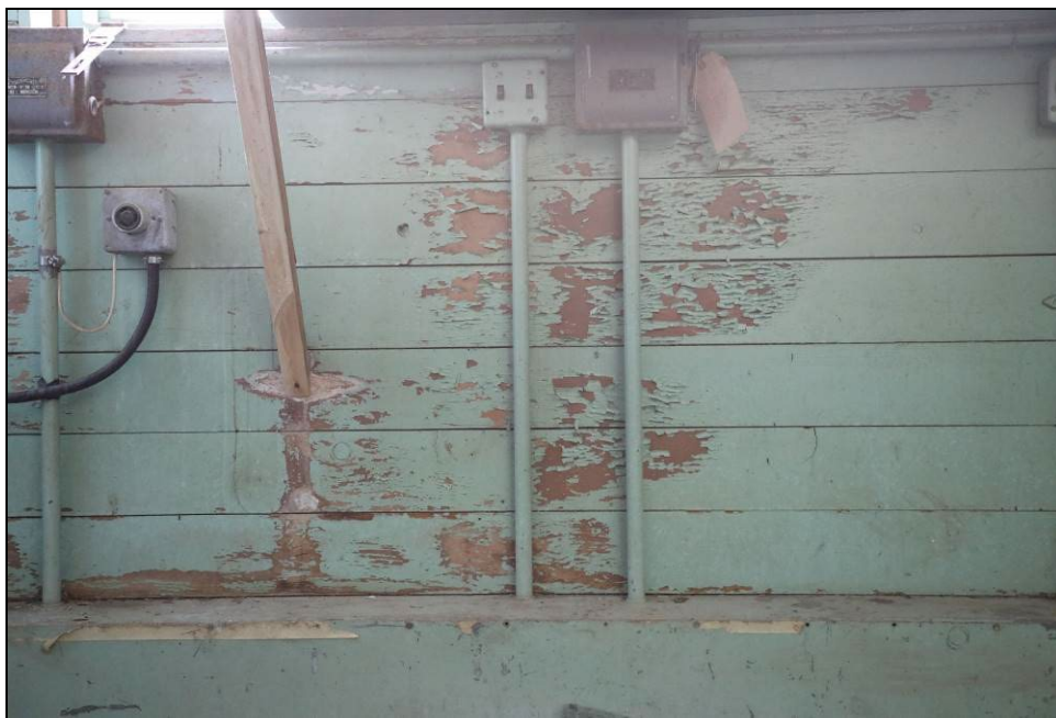
Figure 28. Peeling paint on an interior wood surface.
