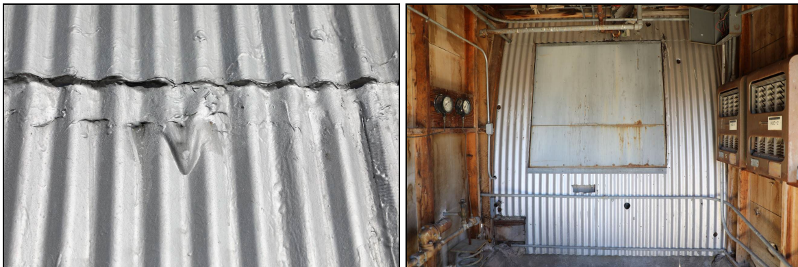
Figure 197. The photo on the left gives an example of the state of the top coat, while the photo on the right shows an original finish section that will help with researching the correct application.
