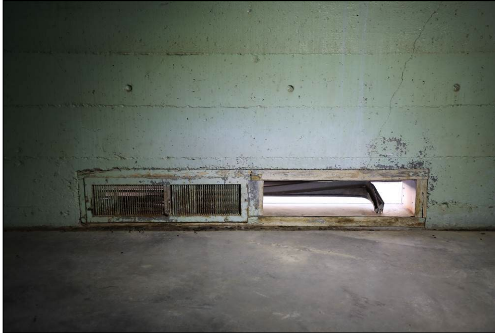
Figure 14. The vent cover is missing and needs replacing.
