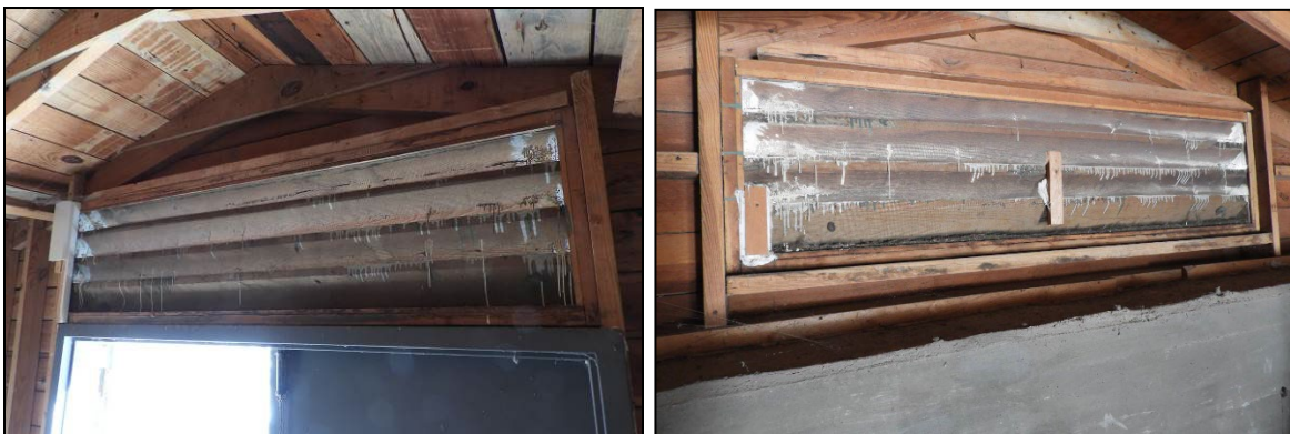
Figure 152. The interior screens over the louvered vents require maintenance.
