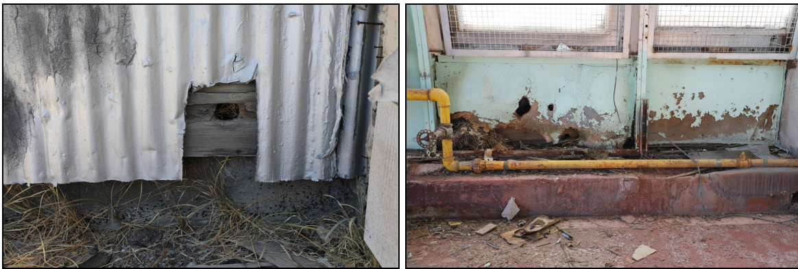
Figure 198. Just two examples of the types of holes found throughout the building.
