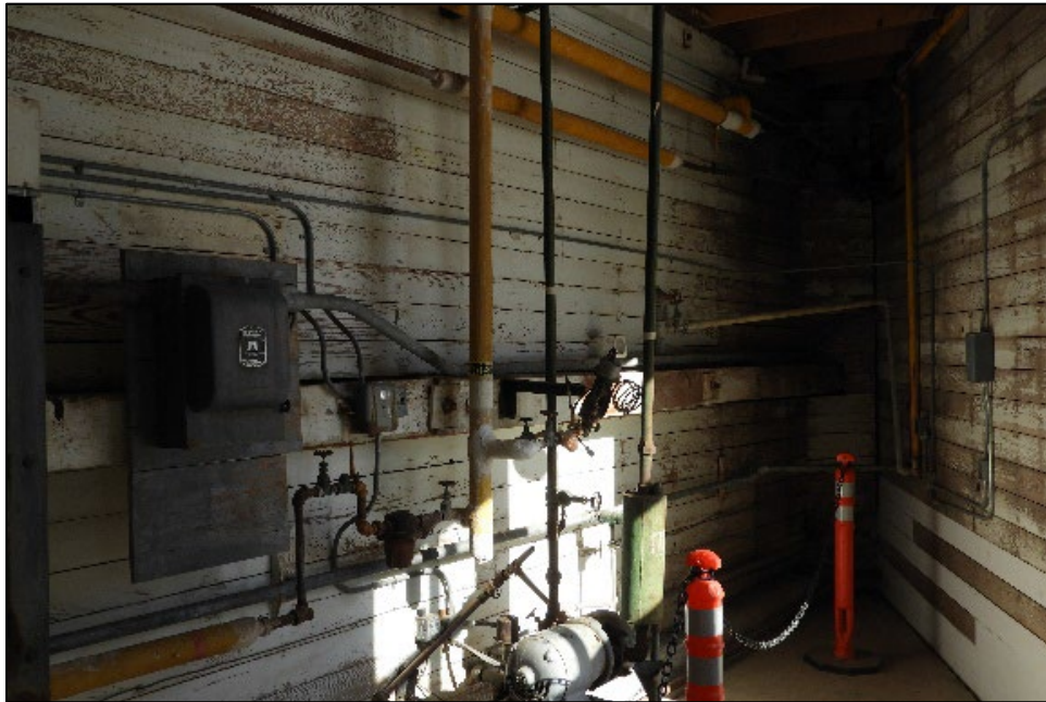
Figure 119. Paint has worn off considerably.
