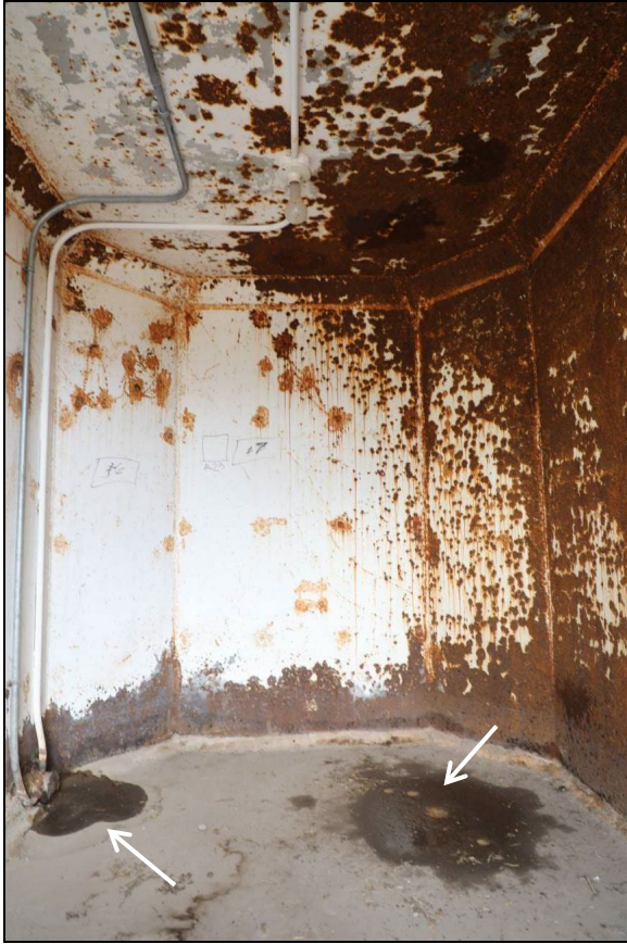
Figure 175. Photographs show active leaks and standing water on the roof.
