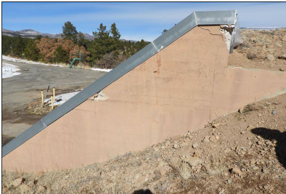
Figure 52. Photo shows the missing corner along with cracking and other issues.
