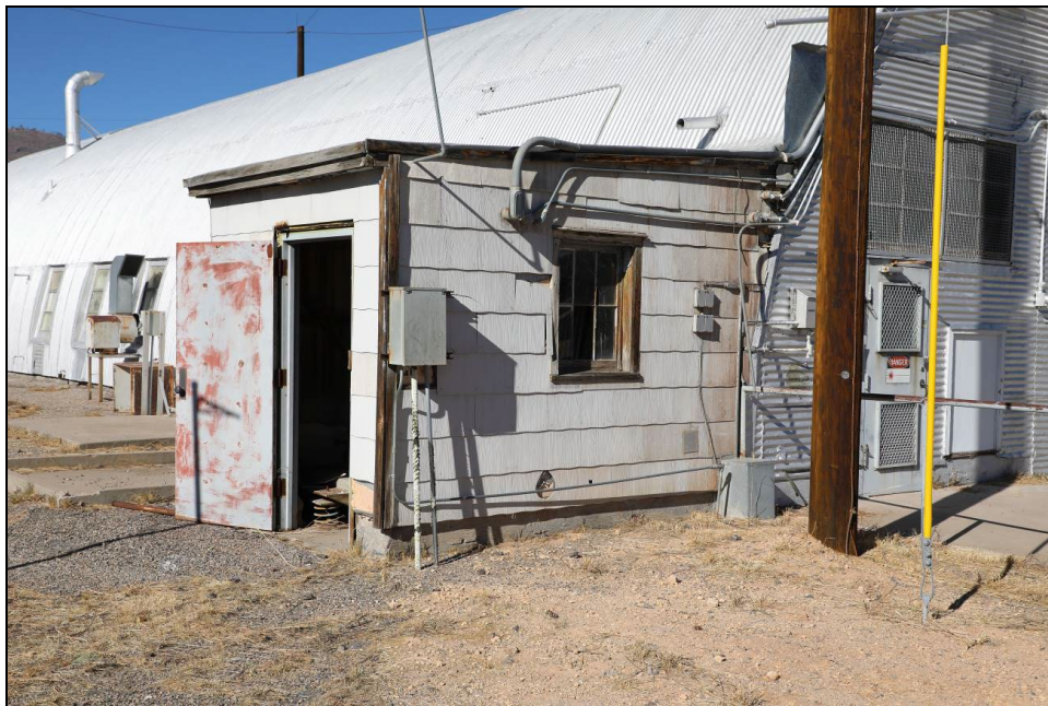
Figure 205. The eaves above the door can be seen here as weathered and lacking paint.
