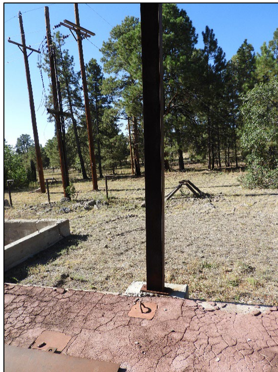
Figure 87. The beam does not make sufficient contact with the concrete base underneath it.
