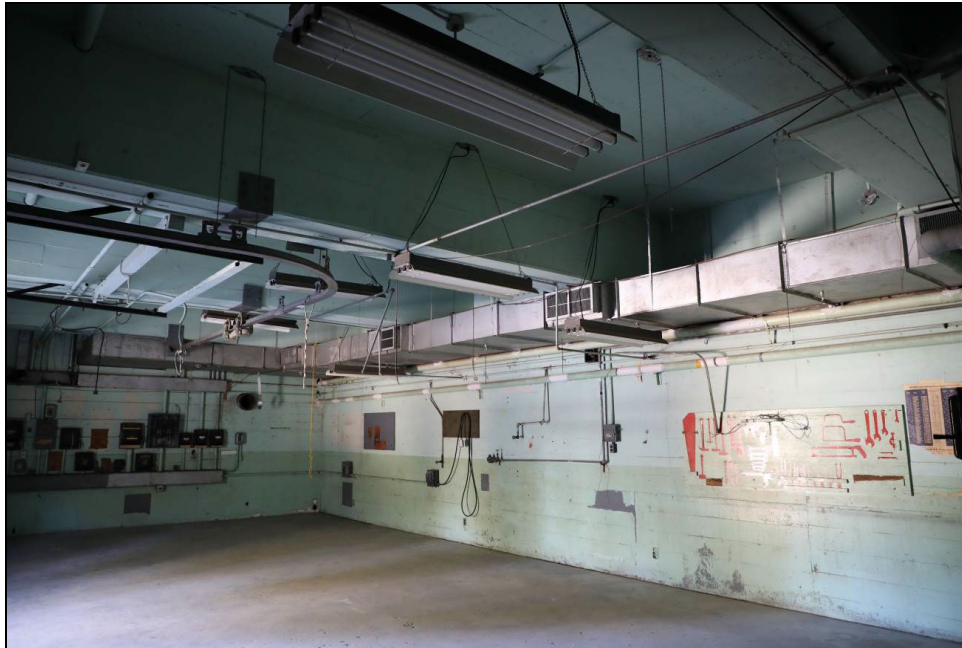
Figure 29. The non-period ductwork stands out in the interior rooms, and also provides a surface for rodent movement.
