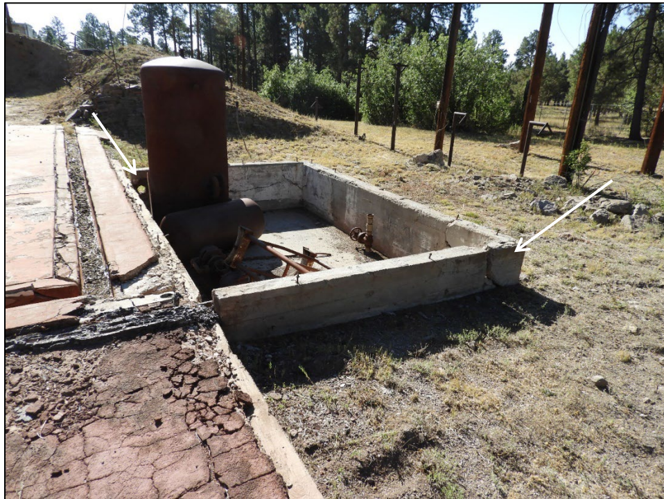
Figure 93. A larger corner separation is evident in the southwest corner and a utility hole can be seen in the northeast corner.
