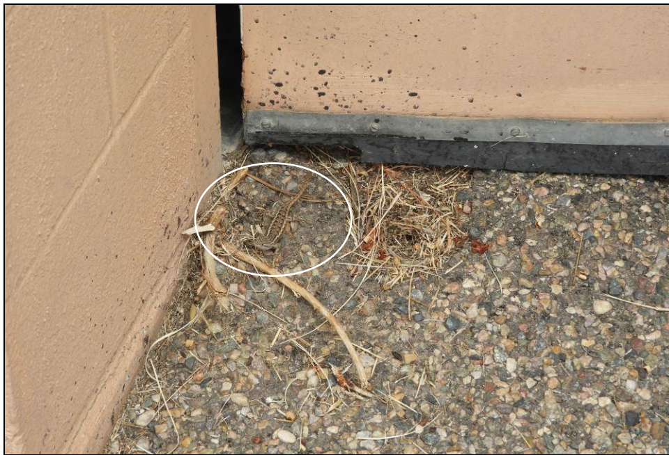
Figure 72. The rubber underside of the door sweep exhibits serious deterioration and allows passage of pests from the exterior to the interior.
