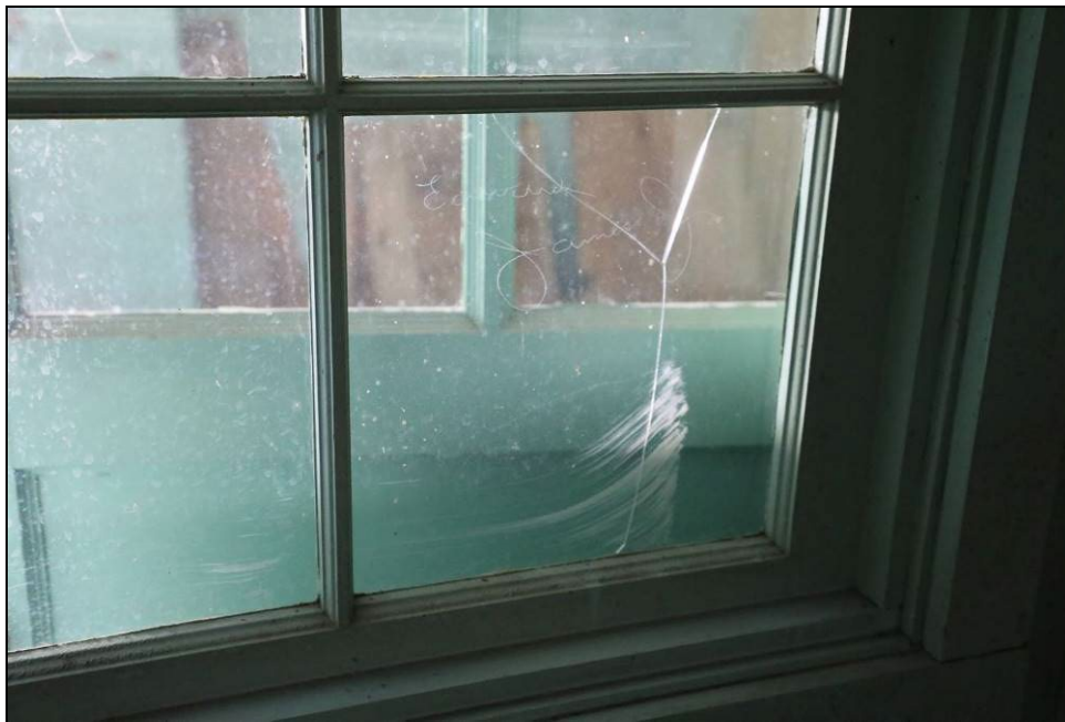
Figure 25. View from the interior of the cracked glass pane with etching.
