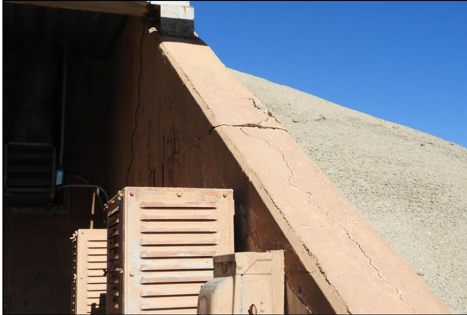
Figure 66. Significant cracking can be seen on the cap of the east wing wall.
