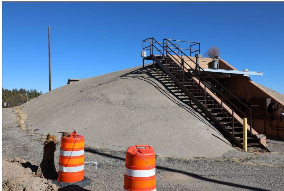
Figure 74. The parging over the earthen berm extends from the sides and back of 11-0003 to the back and sides of 11-0002.
