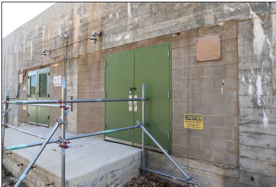
Figure 38. The non-original concrete block can be seen here around the green double doors.
