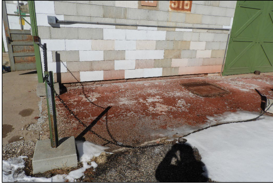
Figure 112. The Hubbelite separation is considerable and likely irreversible.
