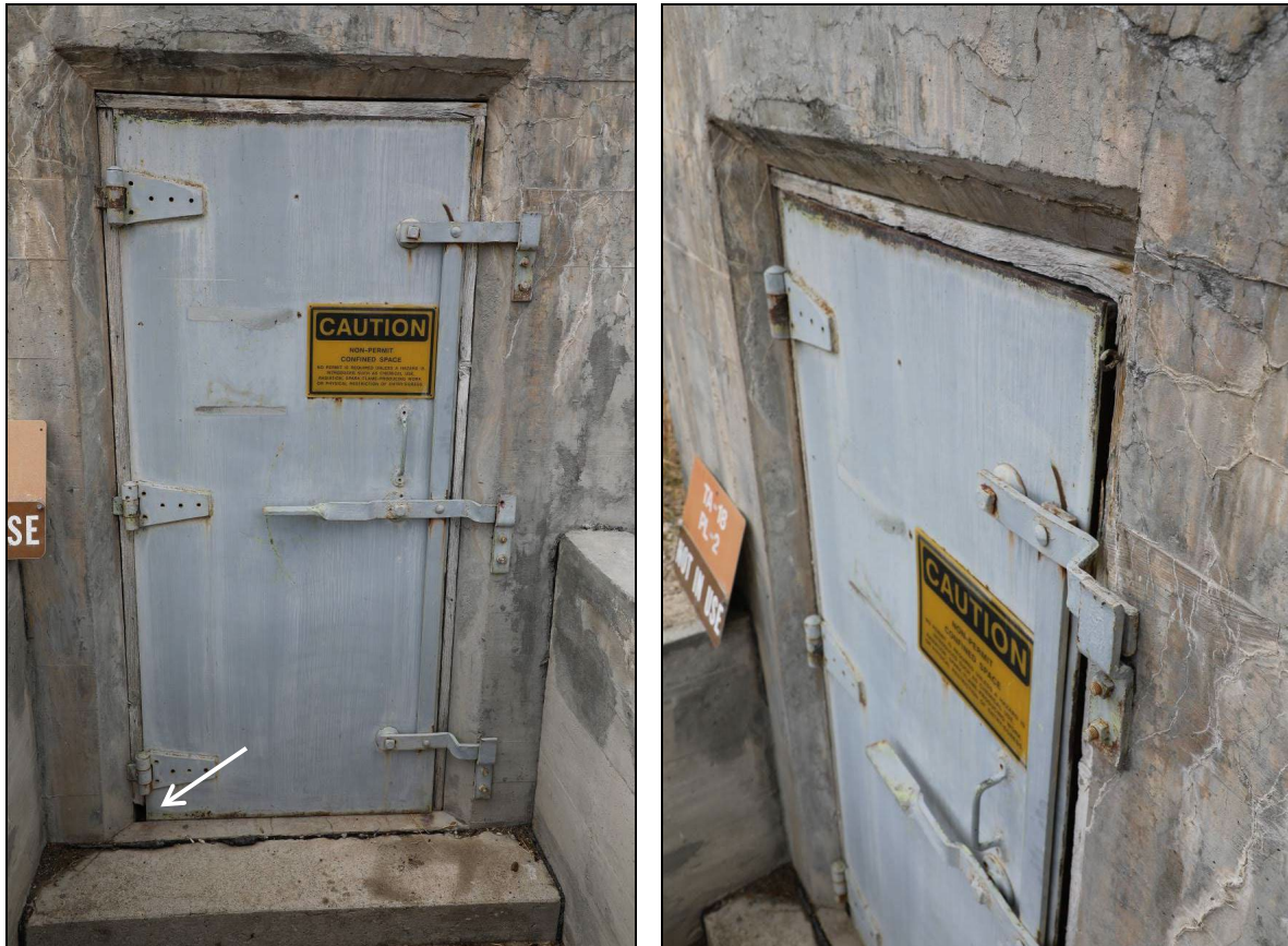
Figure 168. Photos showing the condition of the entrance door frame.
