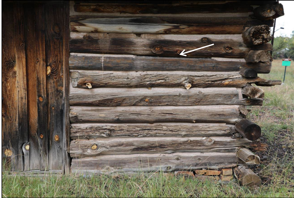
Figure 184. Daubing has also eroded from this area.
