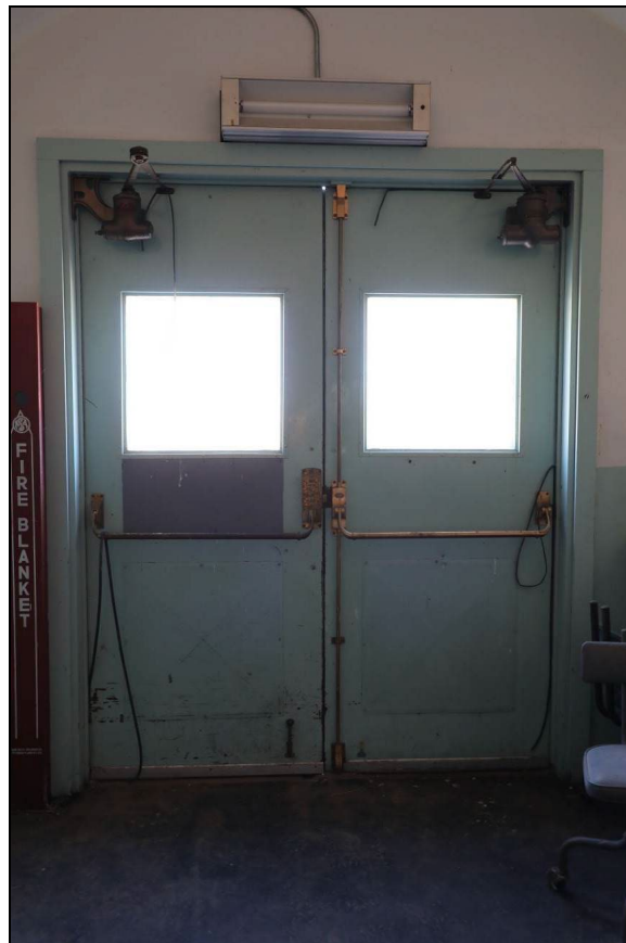
Figure 200. Example of a door opening with some problems - repainting is needed, weather stripping is sagging, and the operability is problematic.
