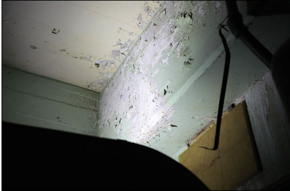
Figure 27. Peeling paint on and near the concrete ceiling.
