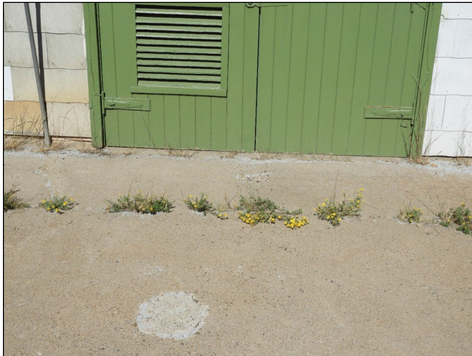
Figure 121. Damage is starting to occur at the base of both doors due moisture penetrating the bottom of the doors.
