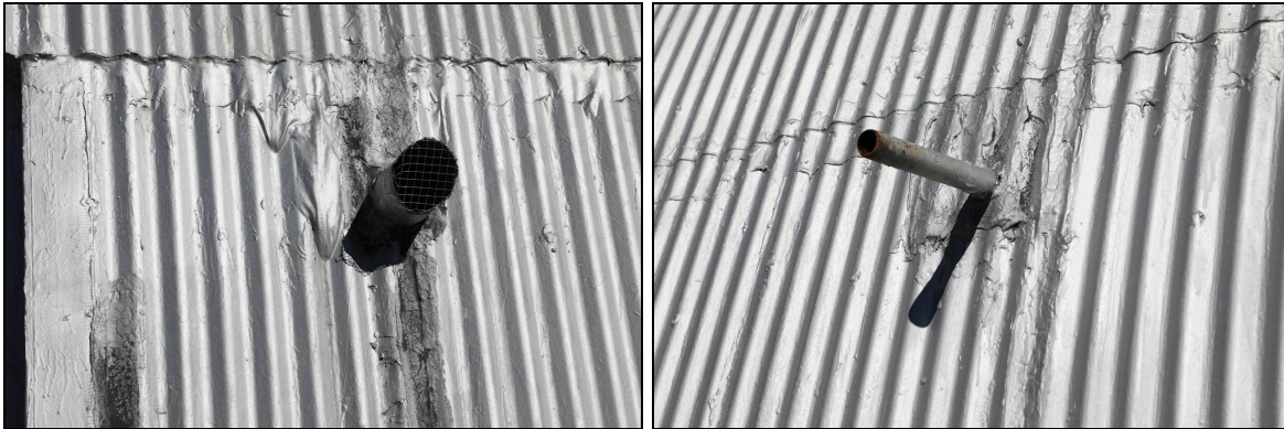
Figure 199. Photo shows two examples of pipe ends needing new screen.
