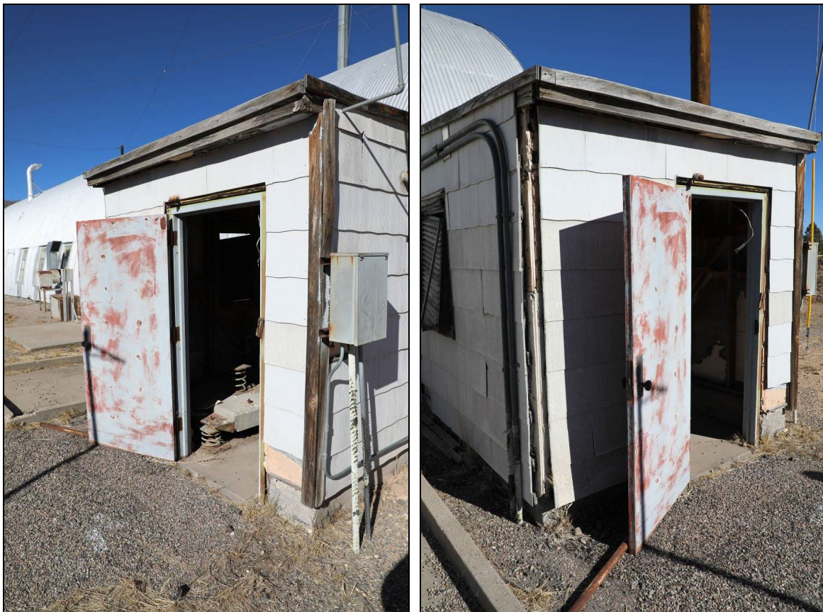
Figure 206. The door trim will require extensive work due to a long period of neglect.
