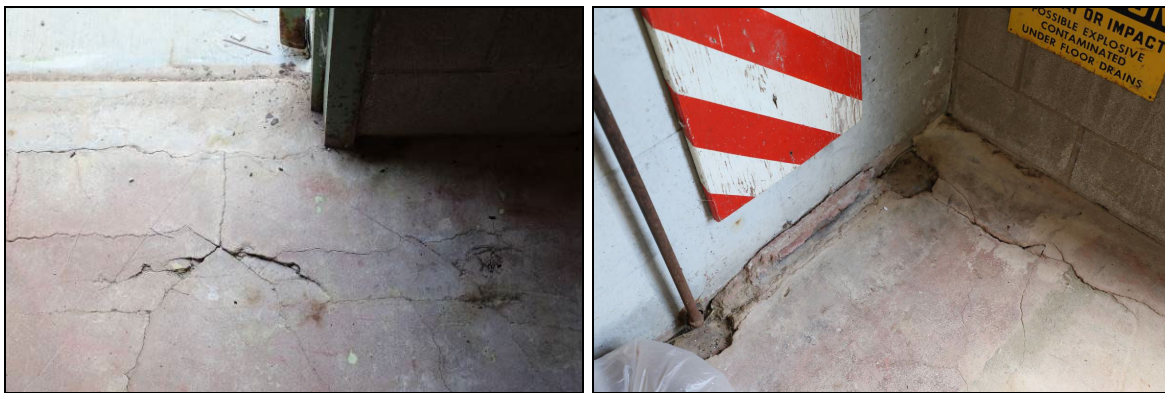
Figure 44. Examples of cracking Hubbelite.
