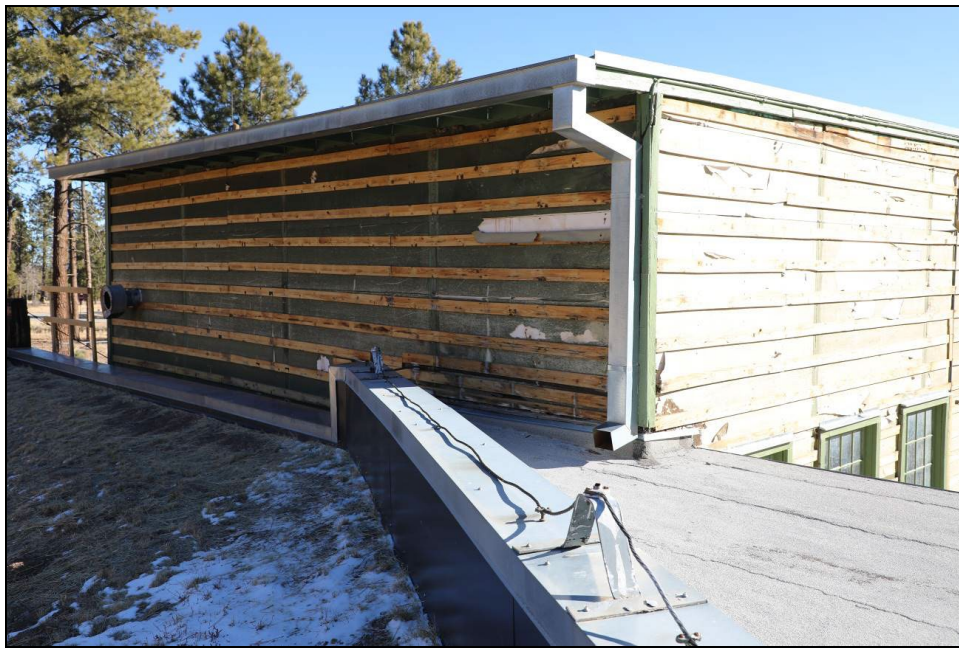
Figure 116. Photograph shows the current gutter and drainage system from the roof of 16-0516 to the roof of 16-0517.
