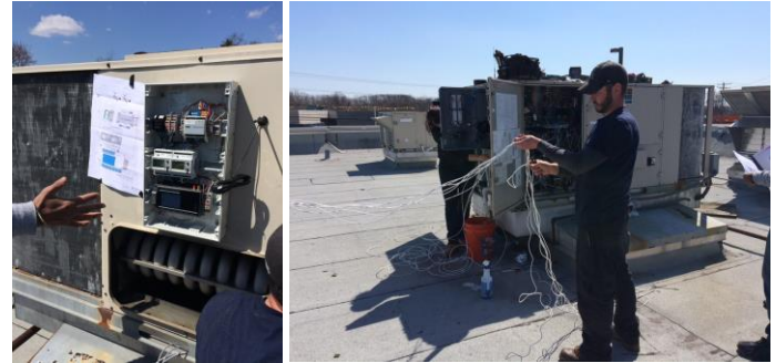
FIGURE 5: A PHOTO OF CLIMACHECK AFDD TOOL INSTALLATION AT CHILI'S IN MILFORD, CT.
