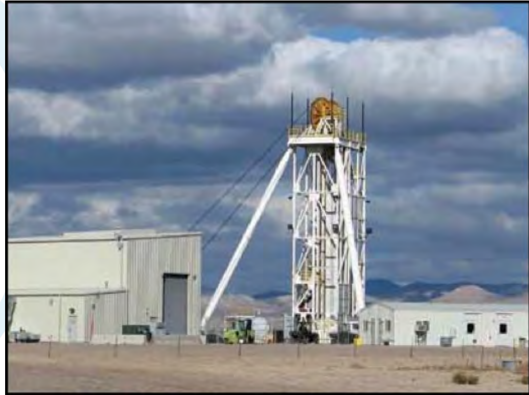
Hoist for personnel, equipment and mining tailings at the surface in Area 1
