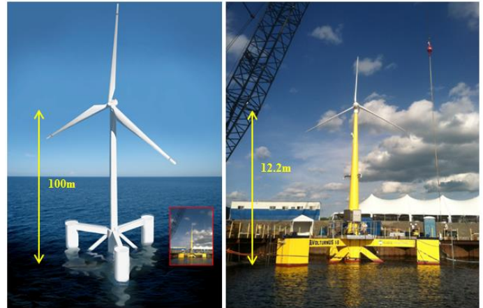
FIGURE 3. (LEFT) VOLTTURNUS 6MW FULL-SCALE DESIGN AND (RIGHT) 1:8 PROTOTYPE DEPLOYED IN JUNE, 2013
