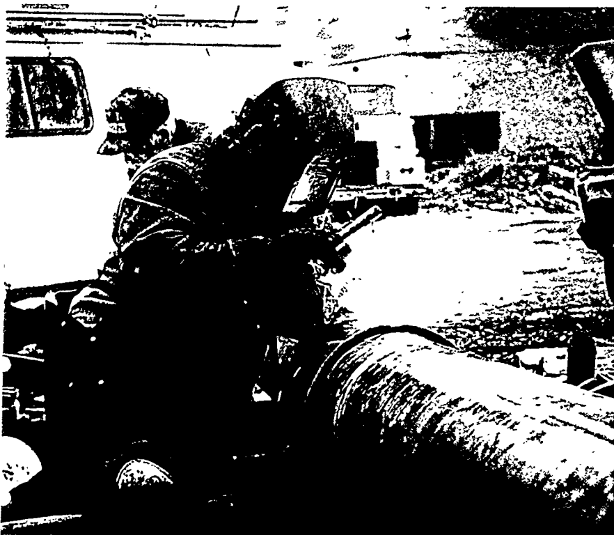
2. TSLJ under construction
