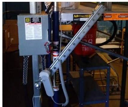
Figure 16. Emergency circuit breaker for tube furnace
