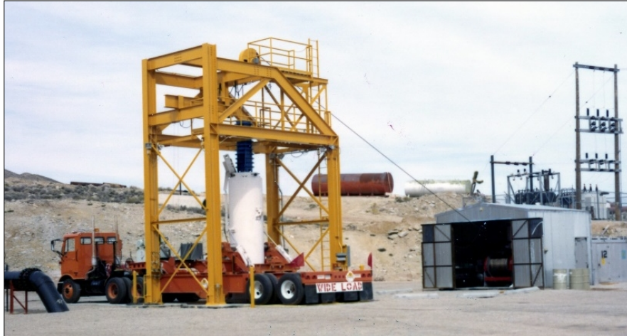
Fig. 4. Waste Package Being Lowered Through Transportation Cask into Climax Mine Borehole.
