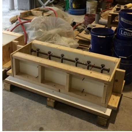
Figure 2.5: Rebar Placed in Formwork Prior to Casting
