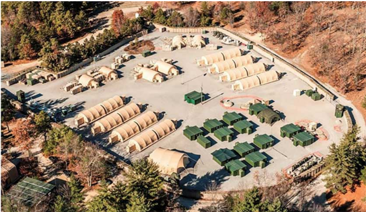
Figure 2. Future Capabilities Integration Lab at Fort Devens, Massachusetts represents two 150-soldier Force Provider Expeditionary basecamp systems developed by the US Army
