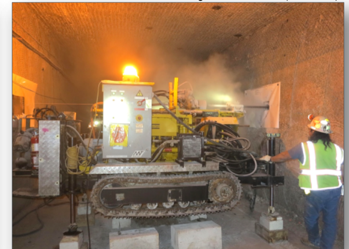
Drilling BATS boreholes (Feb. 2019)
