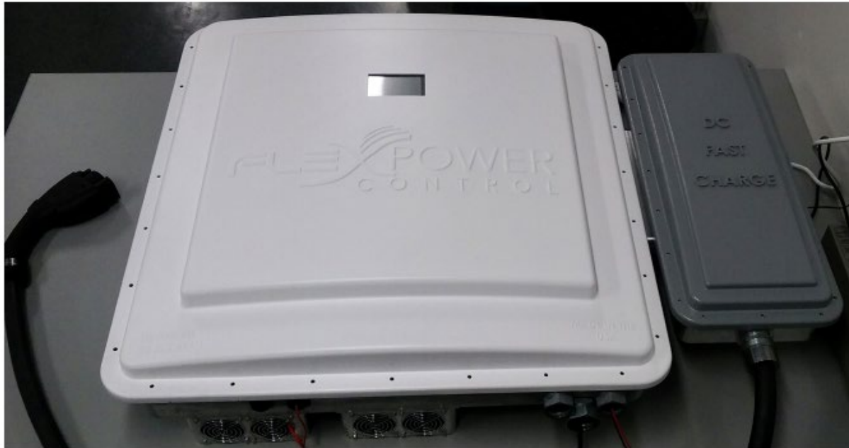
Figure 21 SPIN System Outside View with CCS Cable
