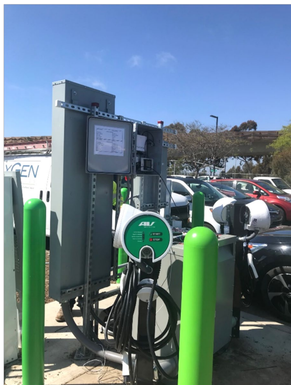
Figure 9: Demonstration Site Charging Island(4 EVSEs, 75KVA Transformer, 400A Panel, Transformer Management System
