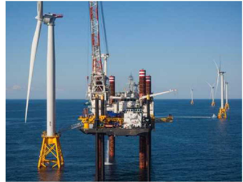
Block Island fixed-bottom wind plant being installed in Rhode Island, the only offshore wind plan in the US
