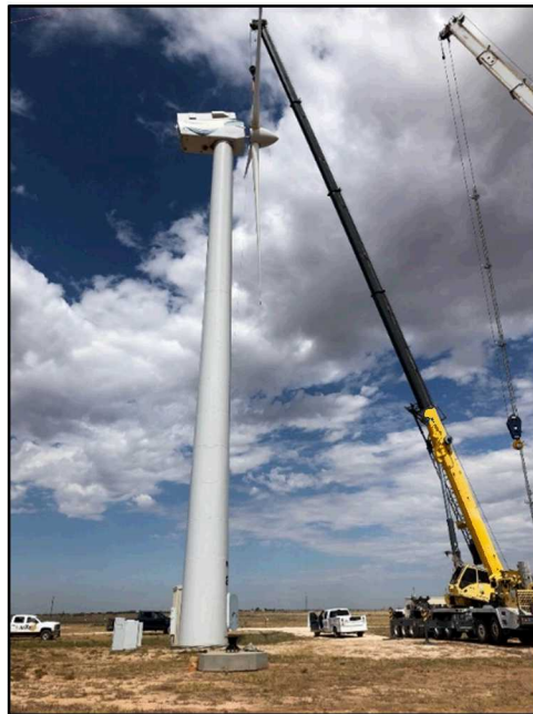
Figure 11. SWiFT Facility rotor installation (Riley, 2020).
