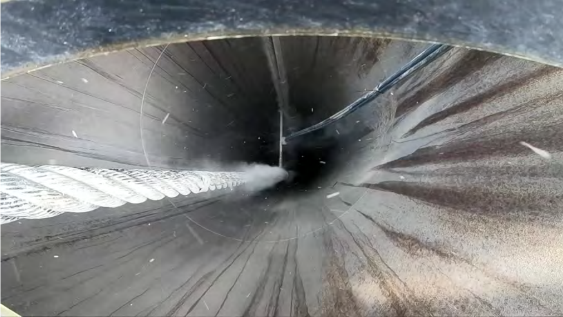
Figure 2. DAG-1 cable cutters from a GoPro directed down the U2ez hole; dust is launched from the cables when tension is released.
