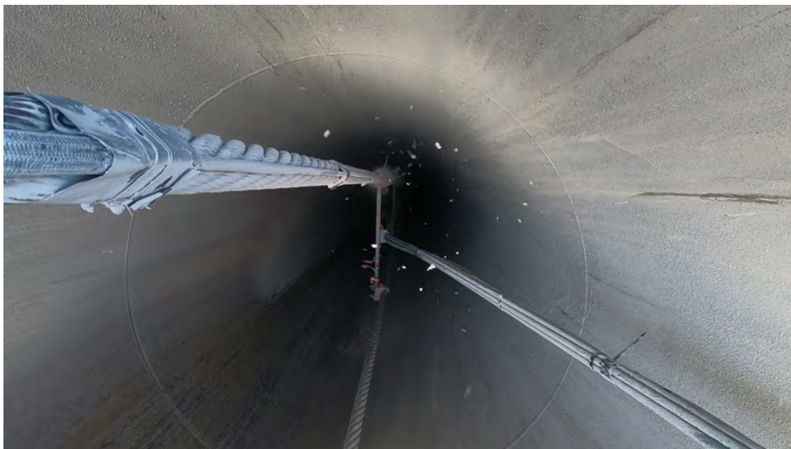
Figure 11. DAG-3 cable cutters from GoPro 2; debris is knocked from the cables when tension is released.
