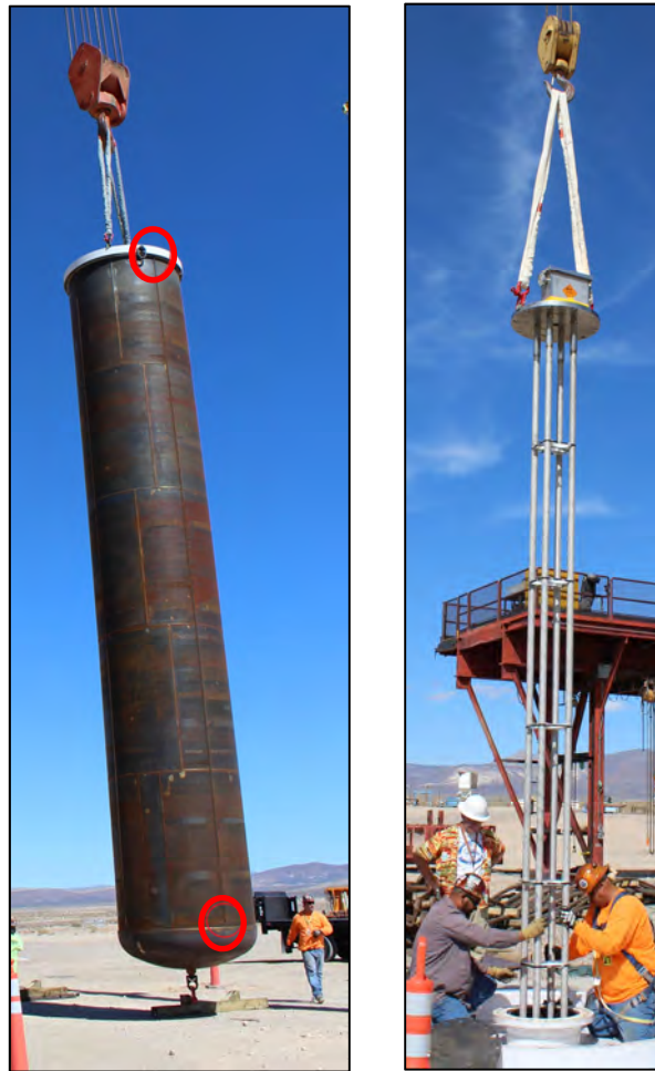
Figure 9 DAG-2 Corrtex Installation
