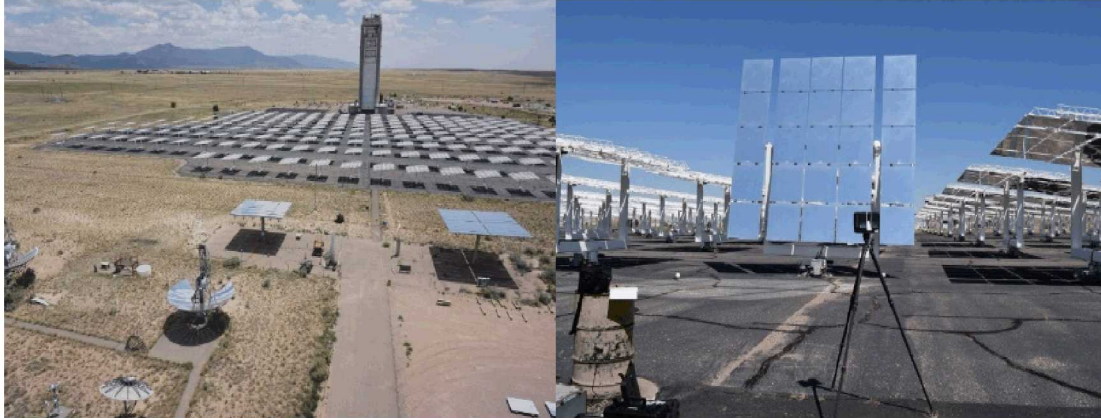
Figure 1 Sandia NSTTF solar tower and the heliostat field (left) and an NSTTF heliostat with 3D LiDAR Scanner
