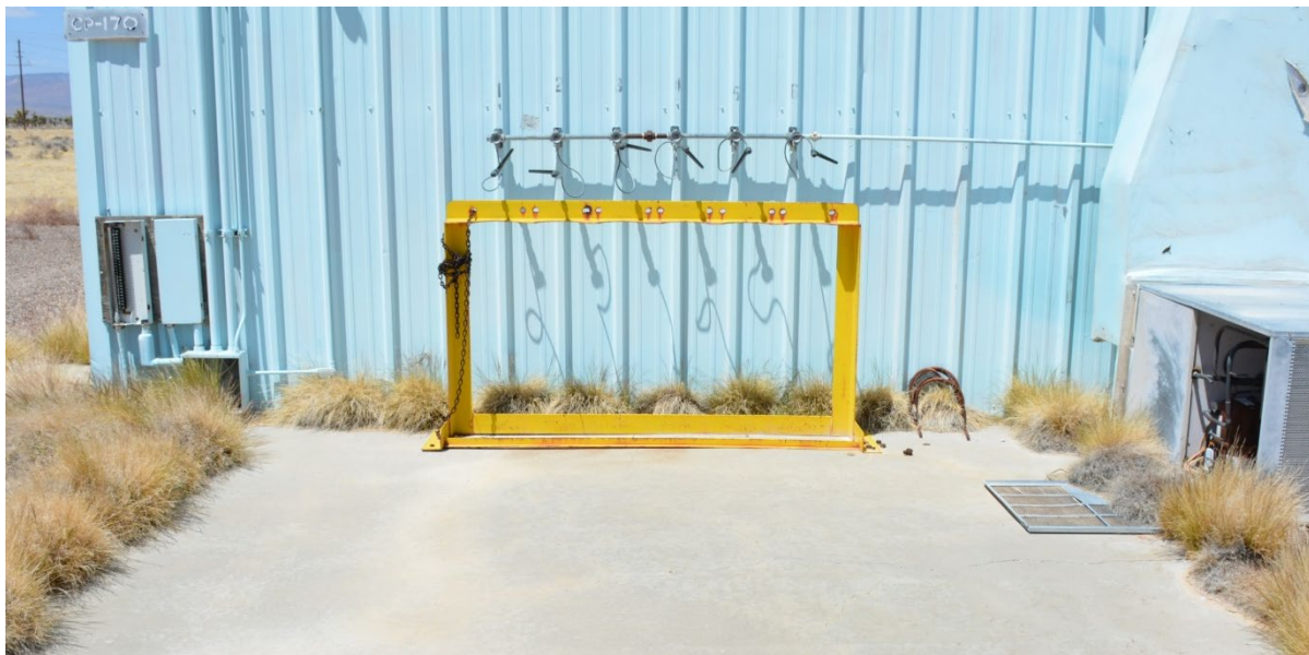
Figure 10. Filling station for weather balloons on the south side of Building 06-CP-170, facing north (DRI DSC_2985, 2021).
