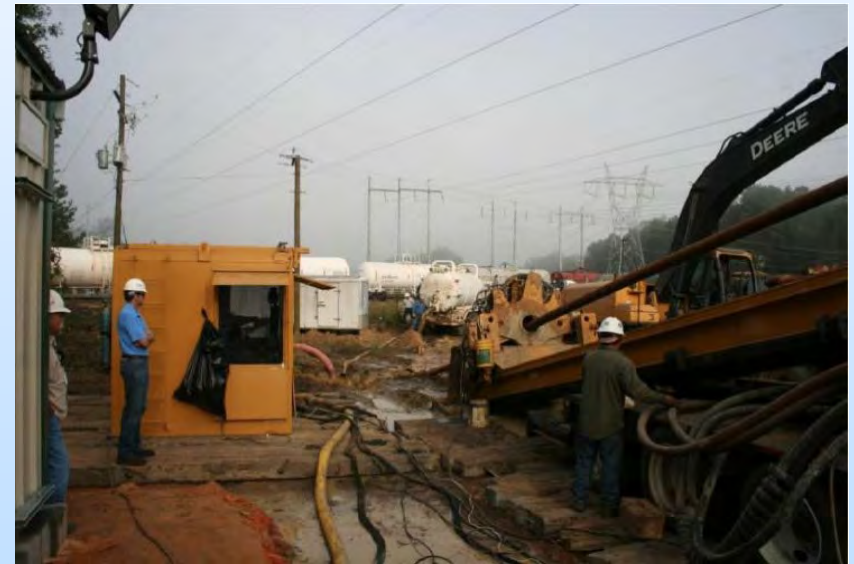
Horizontal Directional Drilling under Alabama Highway U.S. Route 43.
