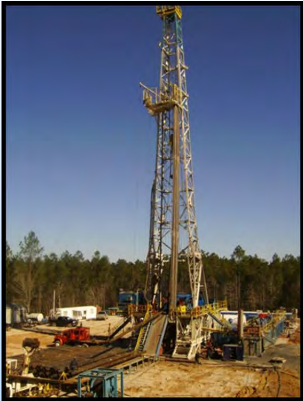
Installation of Injection Well D9-7 #2
