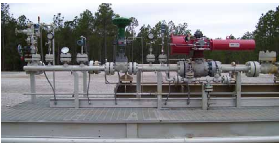
Discharge side of horizontal pump
