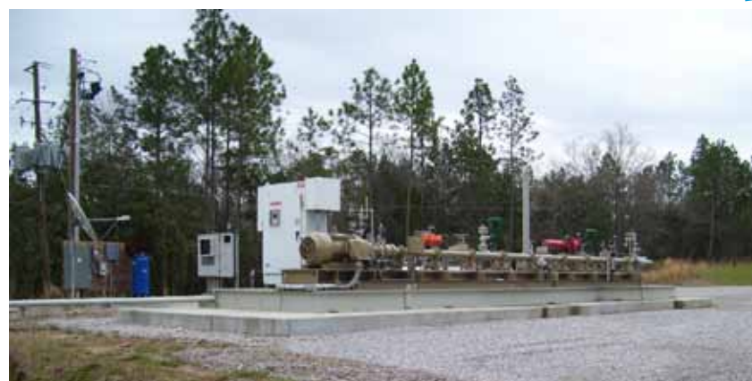
Check meter station to horizontal pump
