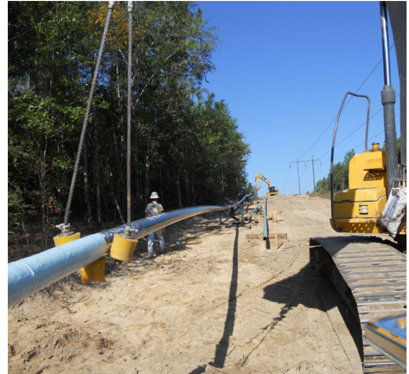
Handling pipe for horizontal directional drill
