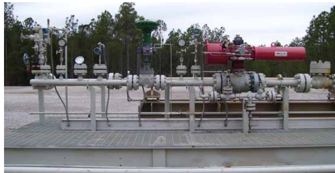
Discharge side of horizontal pump
