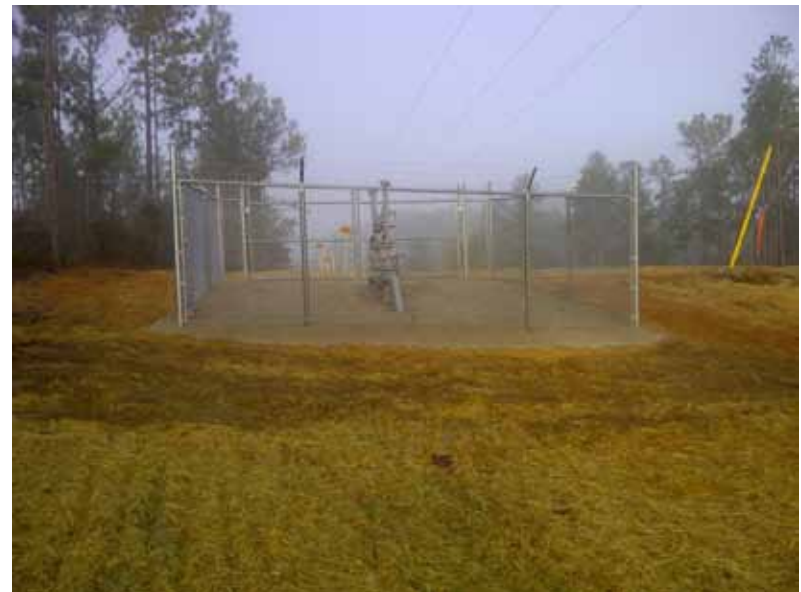
Mainline valve station & CP test station
