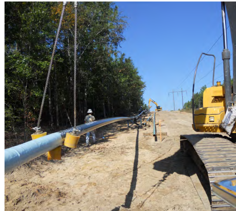
Handling pipe for horizontal directional drill
