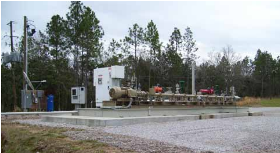
Check meter station to horizontal pump
