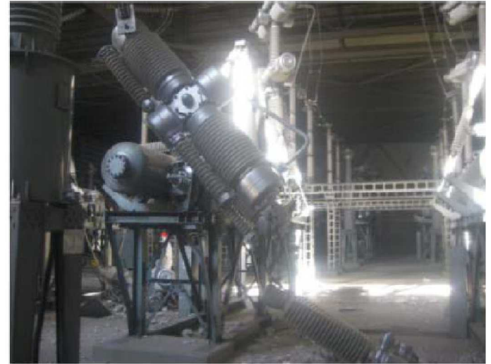
Circuit Breaker damaged
