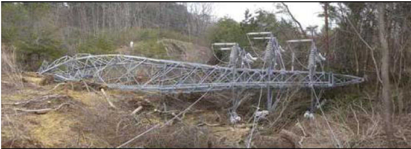
Collapsed tower
