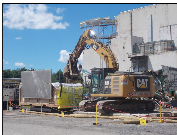
Waste loading with shielding for worker protection
