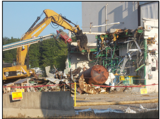
MPPB Utility Room (UR) demolition in progress
