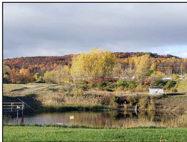
Controlled SPDES discharges occur from Lagoon 3
