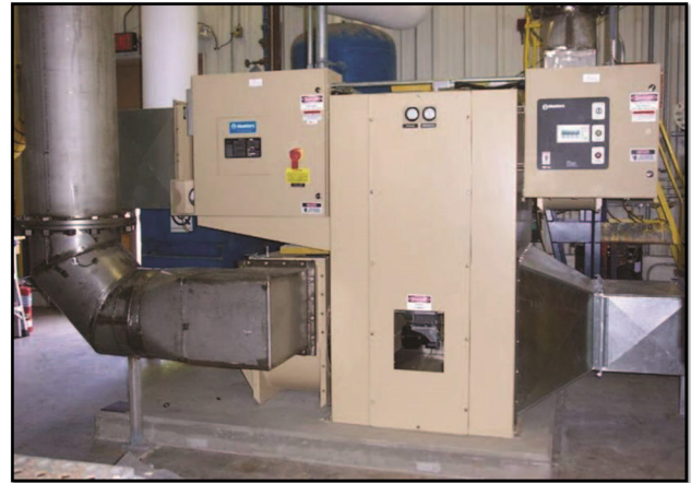
The Tank and Vault Drying System (T&VDS) exhausts through the Supernatant Treatment System (STS) stack
