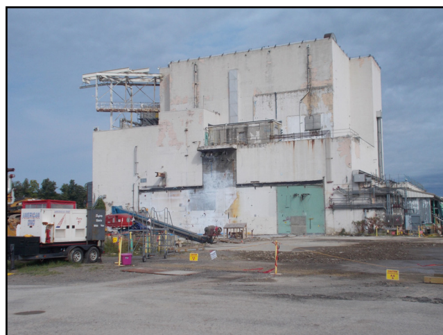
Utility Room (UR) after demolition
