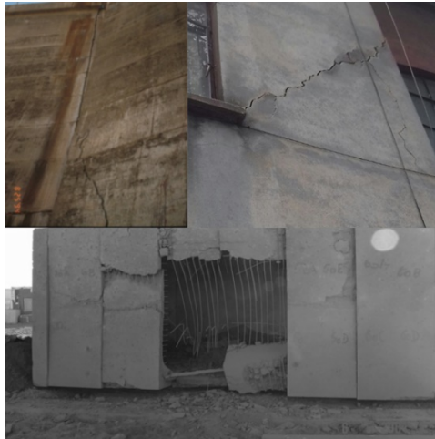
Figure 1-1. (top left) Fracture in the Pacoima Dam during Northridge Earthquake [3], (top right) External damage of a concrete building following the 7.1 Magnitude earthquake in Mexico City on Sept. 19, 2017 (Buchanan, Lee, Pecanha, and Lai, The New York Times, 2017), (bottom) Breaching failure due to a close-in explosion of 6000 kg TNT equivalent [4]
