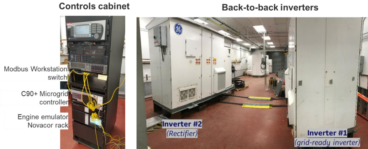
Figure 97: Fully installed and configured PHIL testbed
