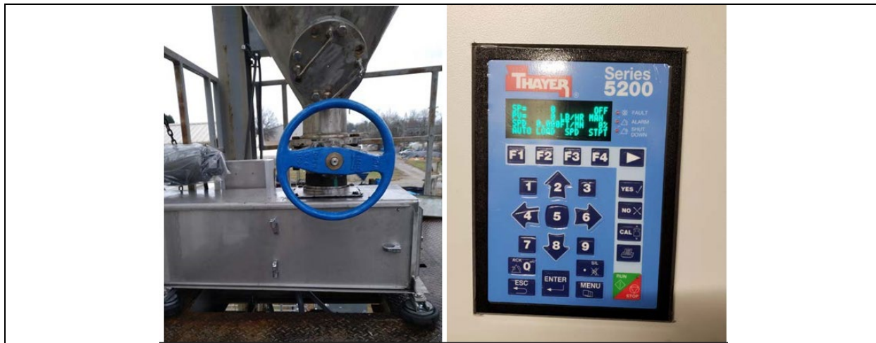
Exhibit 27. Thayer weight belt unit installed (left) and local control unit (right).
