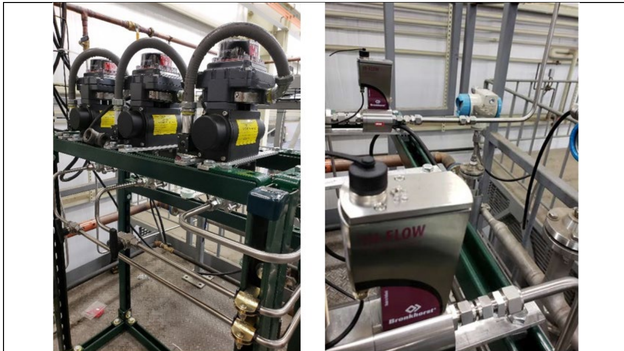
Exhibit 26. Valves for oxygen, nitrogen and natural gas to fifth burner (left) and the associated MFCs (right).
