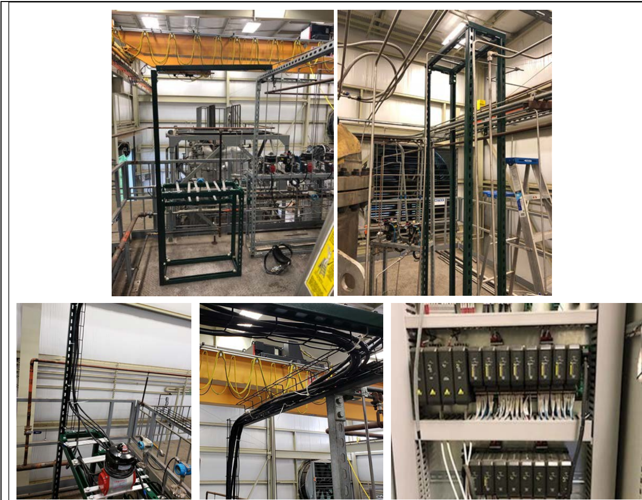
Exhibit 23. Framing and support structures for fifth burner instrumentation (top) and cables and tubing from valve to control system (bottom).
