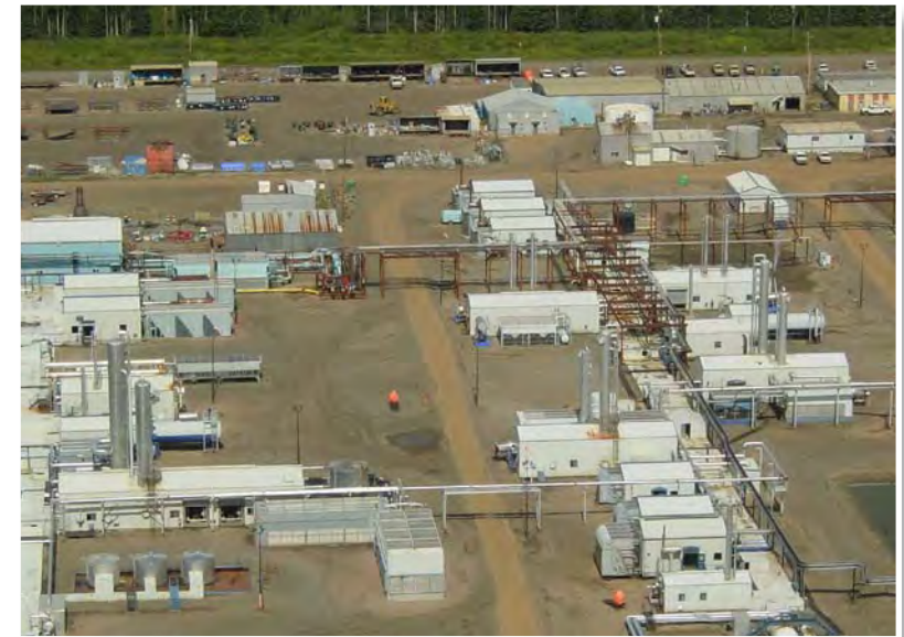
Zama gas plant.
