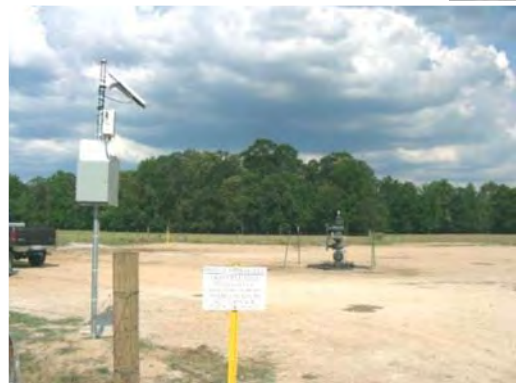
Satellite uplink providing remote access to data collected at the Cranfield dedicated monitoring well.
