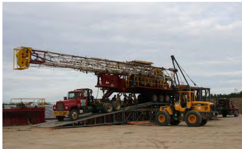
Drilling rig at Mississippi Test Site. (Courtesy of Southern Company)
