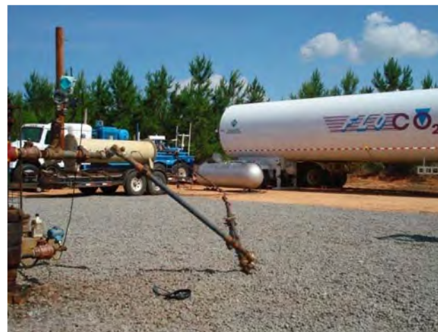
Injection operations at the Black Warrior Basin Coal Seam site near Tuscaloosa, Alabama.
