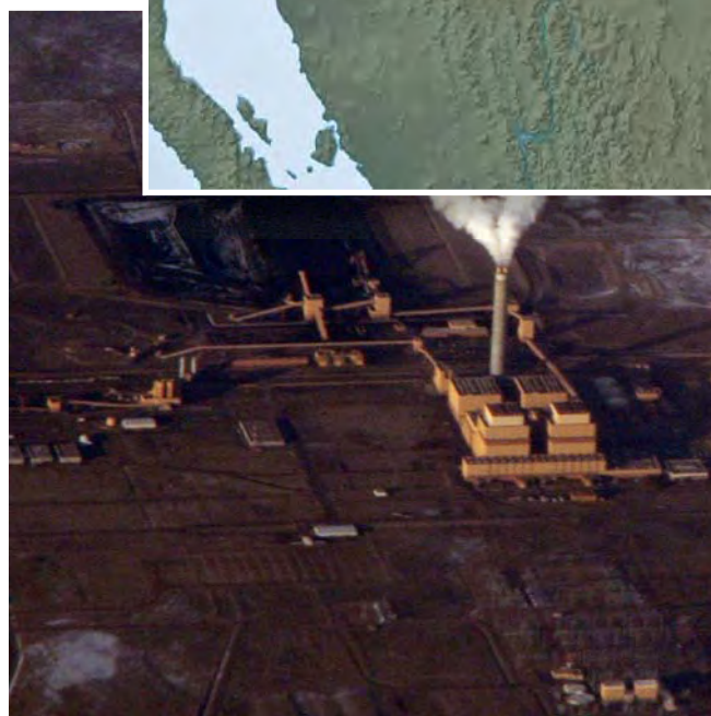
Over 300 electric power plants serve the Southwest region.
