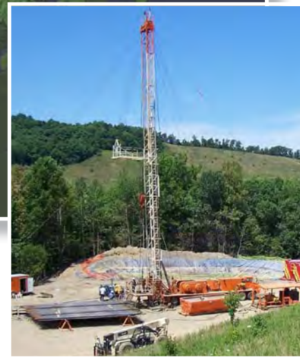
Drilling operations at the Ohio CO 2 storage test well in Tuscarawas County, Ohio. Both CO 2 storage units and natural gas were discovered in this well.
