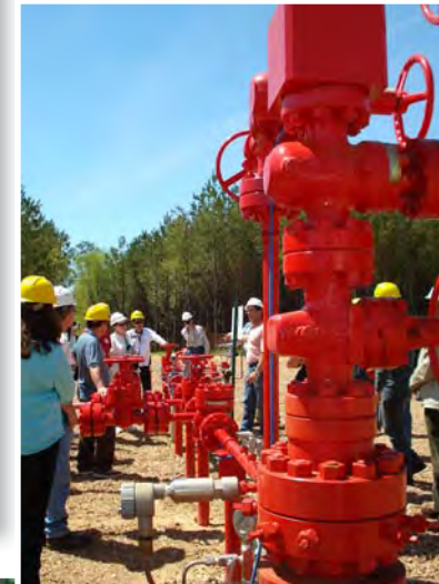
The Development Phase Early Test site in Mississippi (left).
