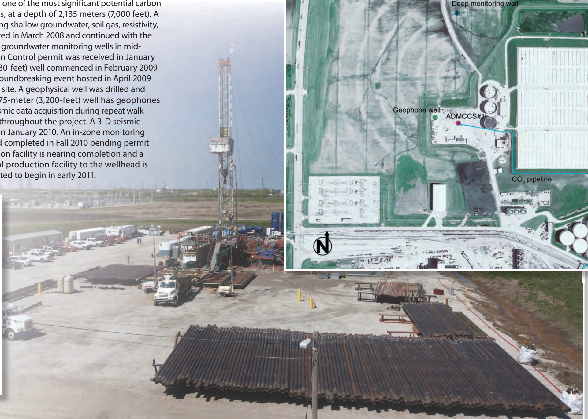
Above: Drilling of injection well at the Illinois Basin—Decatur site; long string casing is in the foreground.
