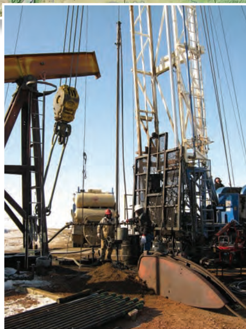
Preparation of the injection well for the huff 'n' puff test.
