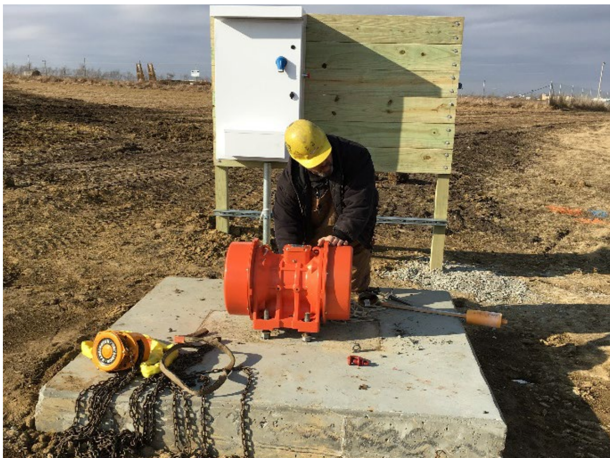
Figure 29. Installed SOV motor and electronic panel.
