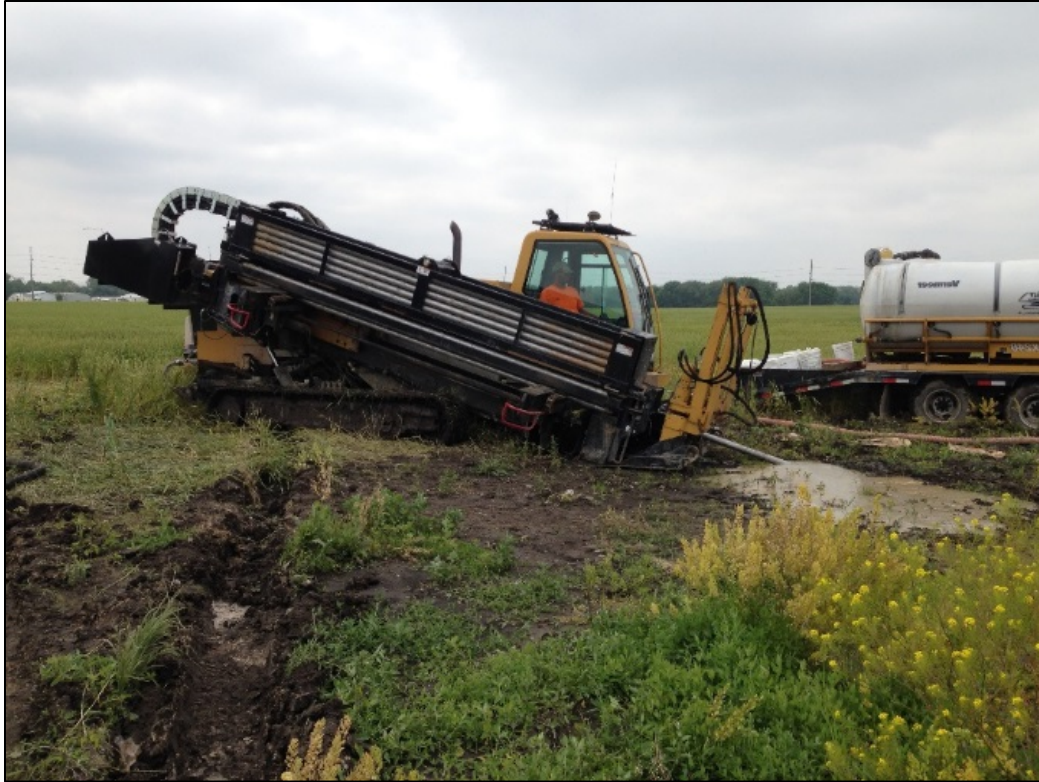
Figure 22. Horizontal directional drilling preparing to install the helical cable.
