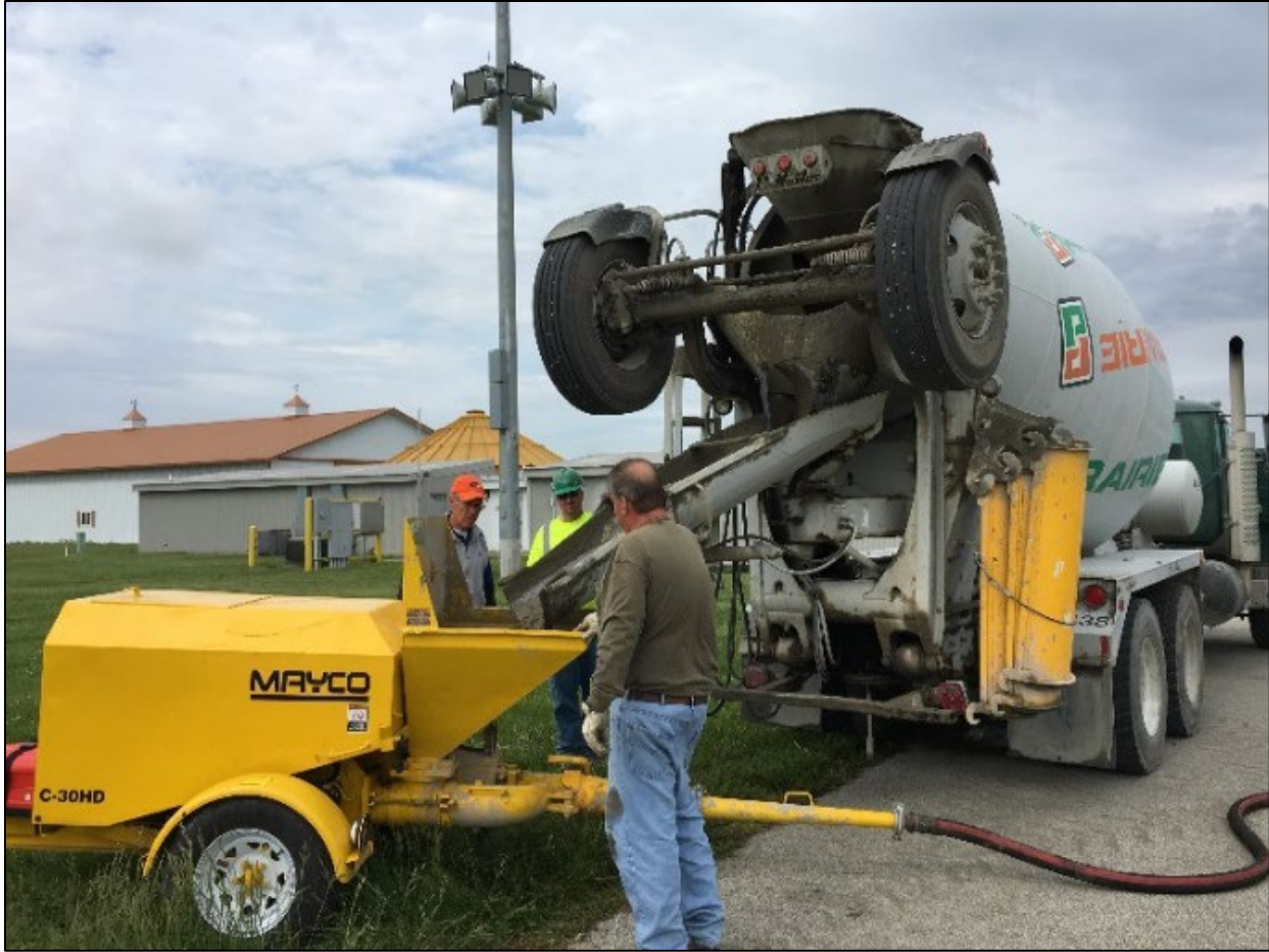
Figure 26. Grouting DAS cable.
