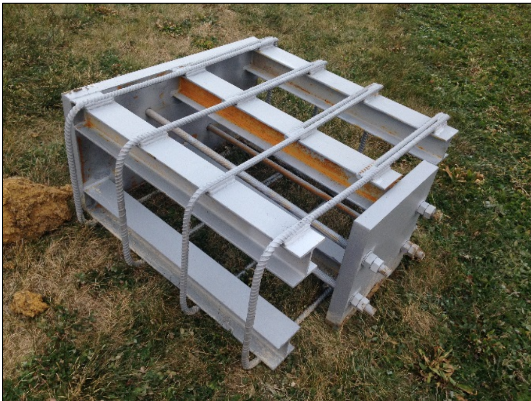
Figure 28. Structural SOV anchor assembly.
