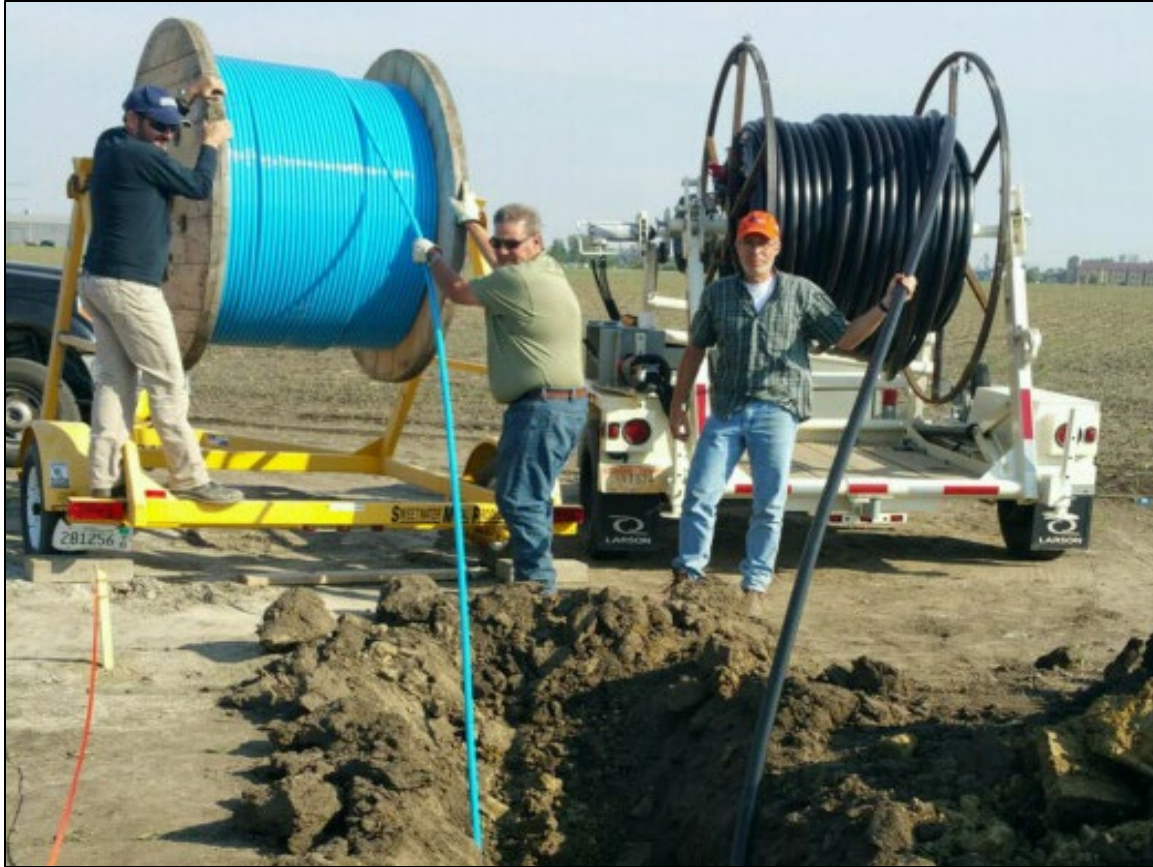
Figure 24. Cable reels feeding DAS cable and grouting conduit into bore hole.
