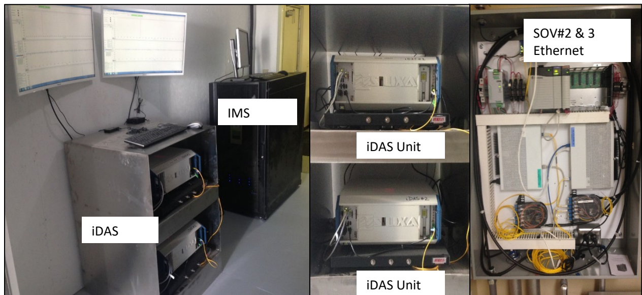
Figure 21. Setup of the IMS Server & iDAS units in the CCS#2 building and SOV#2. On the right, Ethernet switch inside the VW#2 building.
