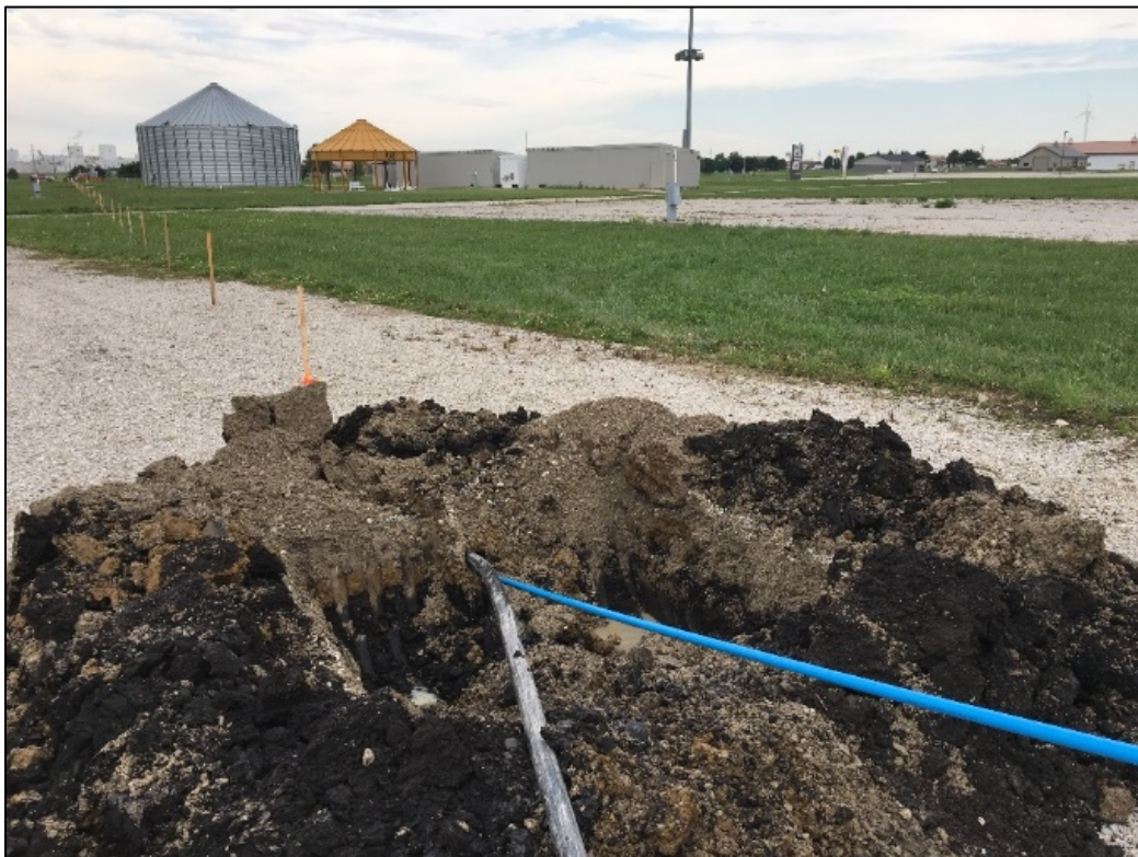
Figure 23. Cable and Conduit pull back.
