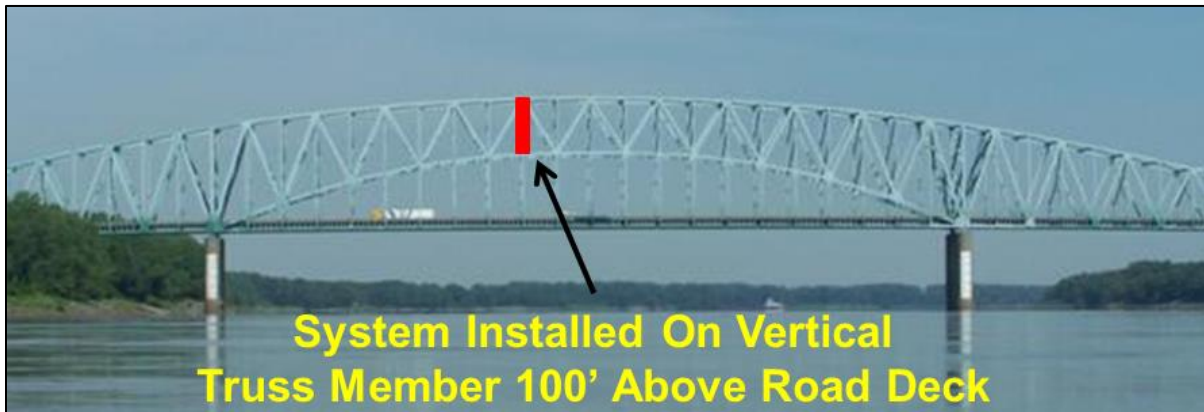
Figure 2-27. Placement of CVM Sensor Network for Monitoring Critical Bridge Welds
