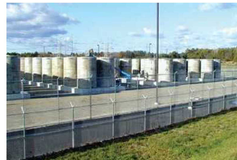
Vertical above grade dry cask storage system at Maine Yankee.
