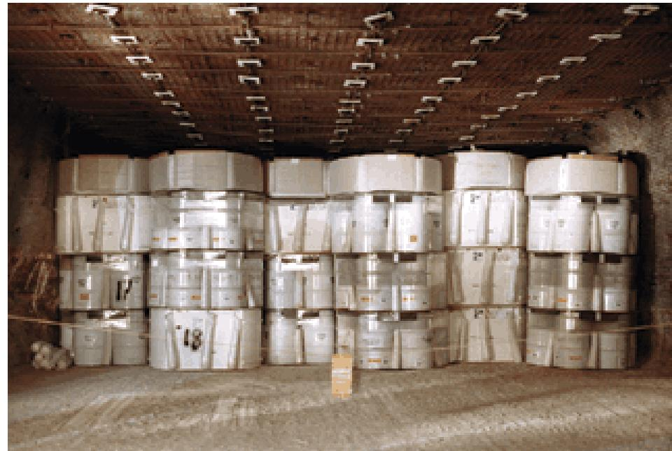
Granular MgO emplaced above waste stacks to consume CO<sub>2</sub> and buffer pH to reduce actinide solubility in brine
