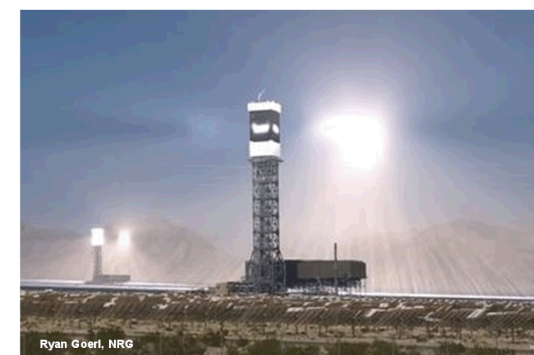
Hot spots caused by standby heliostat aiming strategies that have been reported to singe birds
