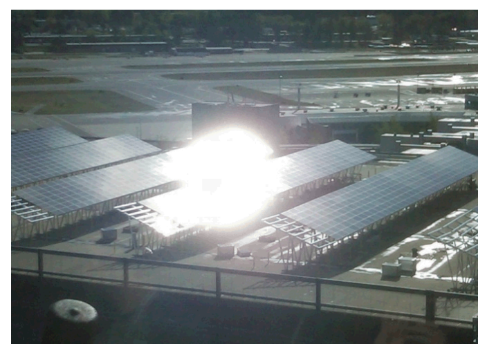
Glare from PV system near air-traffic control tower at Manchester-Boston Regional Airport
