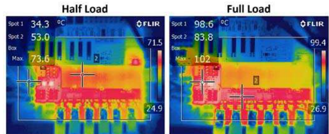
Fig. 26. Thermal images of LLC-DCX at half load (left) and full load (right).
