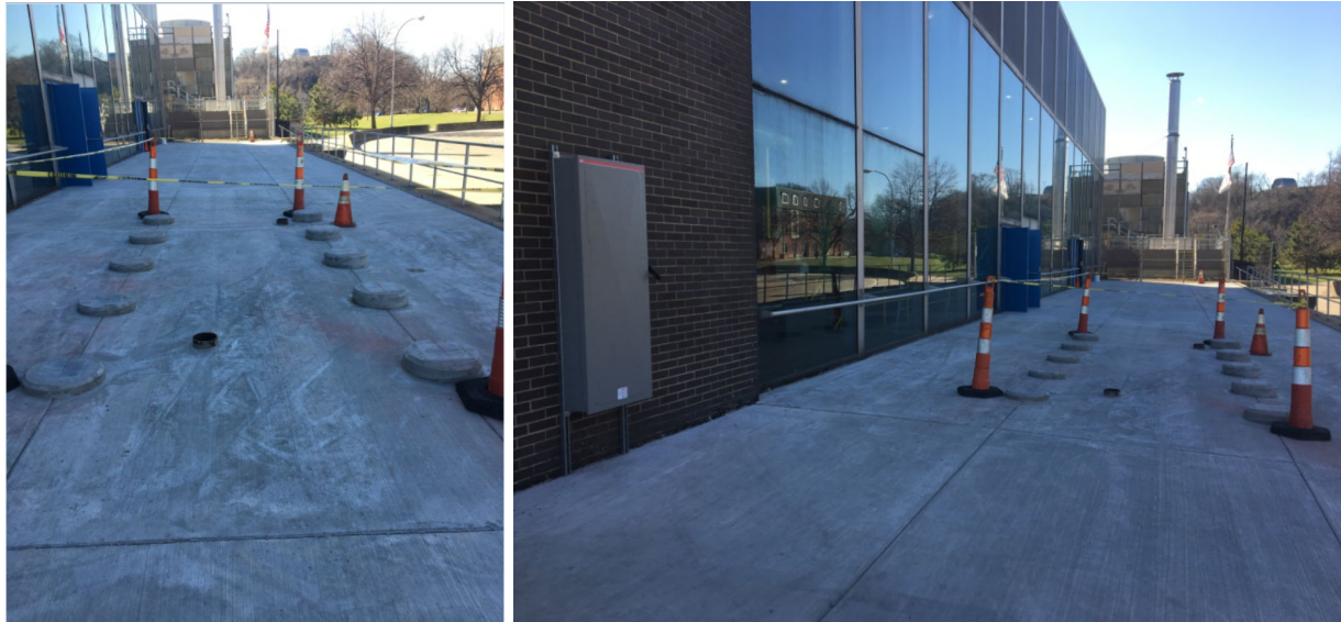
Figure 5-4 New Concrete Upper Deck, Fuel Cell Pier Supports & Pass Throughs
