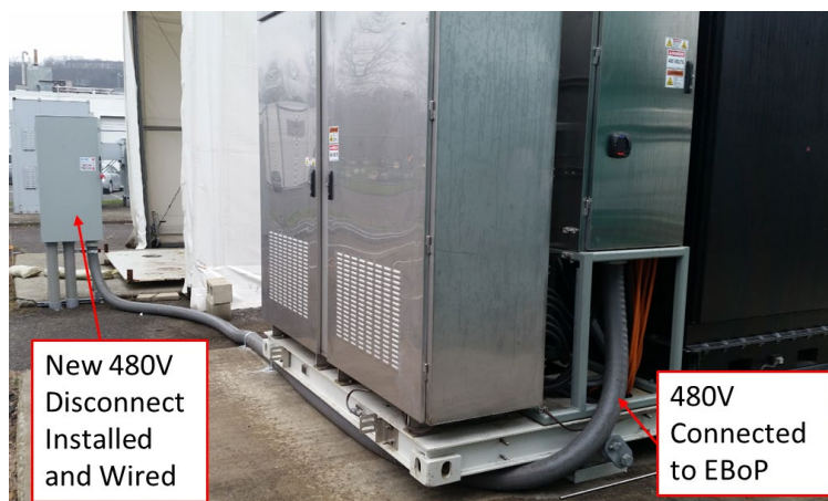
Figure 5-12. 480V Service Installed and Connected to the SOFC Prototype System in Danbury, CT
