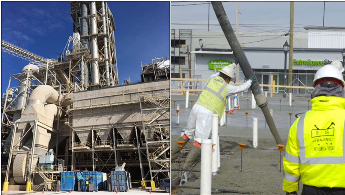
Figure 2. (Left) The CCC-ECL test skids at the Argos cement plant in Calera, Alabama where \text{CO}_2 was captured for utilization in concrete. (Right) Pouring Readymix concrete in Atlanta, GA where CarbonCure utilized the \text{CO}_2 captured at the Roberta Cement Plant.
