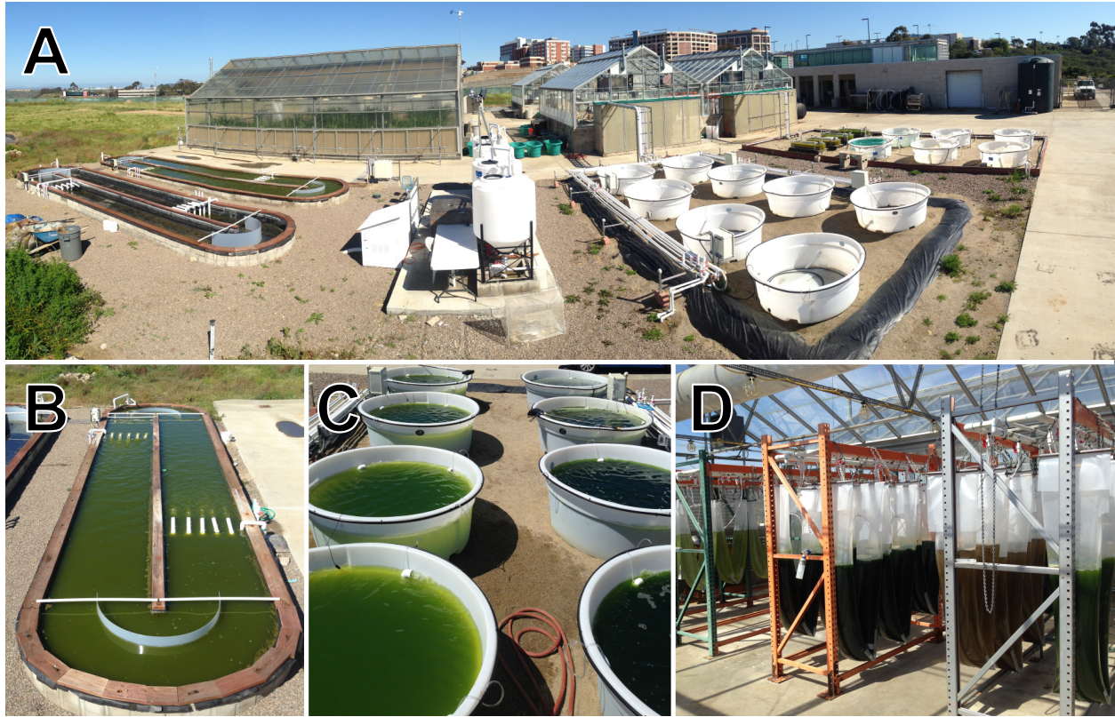
Figure 1. Pilot-scale algae research facility operated by the California Center for Algae Biotechnology (Cal-CAB) at the University of California, San Diego. The half-acre facility (A) is equipped with various cultivations systems located either outdoors (B & C) or in greenhouses (D). This facility has historically been used as an educational platform to study the potential of algae as a biofuel feedstock, including research into algal genetics, dispersal patterns, predator-prey relationships, and biomass productivity.
