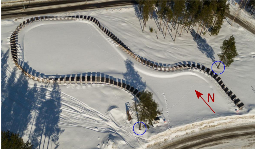
Figure 95: Birds-eye view of the Solvåg solar site in March 2018. The red arrow denotes the North direction, and the blue circles mark trees that have been cut (September 2018) to limit issues with direct shadowing. Photo: Mikael Sundqvist (P-town Productions).
