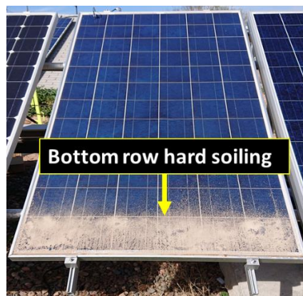
Figure 1-30: Soiling - Manual dusting
