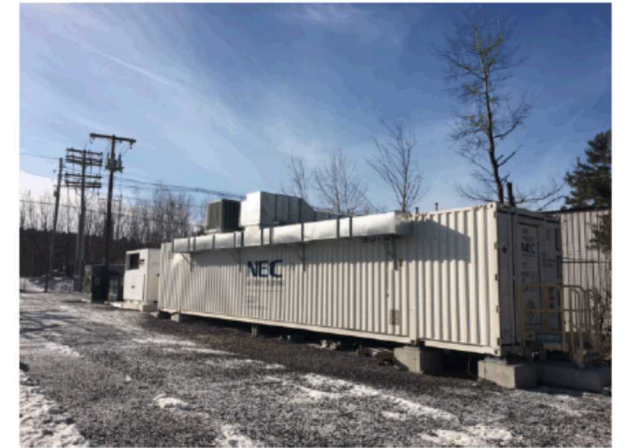
Sterling Municipal Light Department 2 MW, 3.9 MWh system
