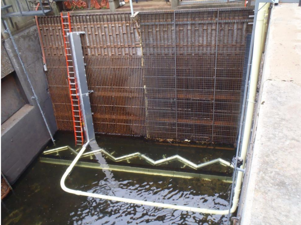
Figure 4-5. Installation of the two eel bypass systems at Mine Falls.
