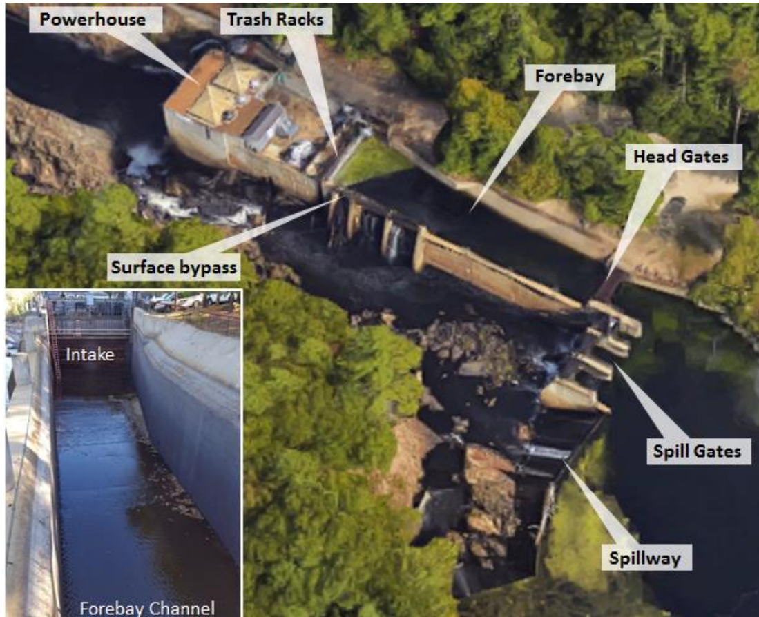
Figure 4-2. Mine Falls Project configuration (inset photo shows dewatered forebay channel with turbine intake at downstream end).
