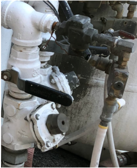
Valve #10 (Energizes Air), fails closed (Fail Safe vs Fail Unsafe). Spring closure
