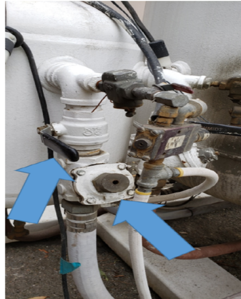
Figure #3 - Choke Valve (Compressed Air Manual Ball Valve) turned off (top arrow) Automatic Air Valve (bottom arrow)
