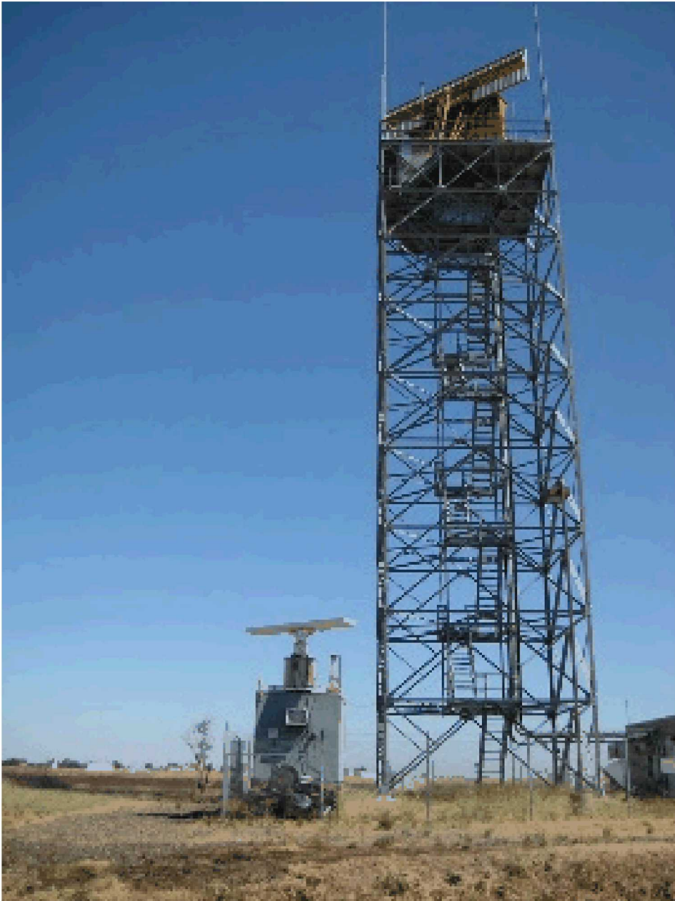
Infill radar (left) next to the DASR tower and antenna on Travis AFB.
