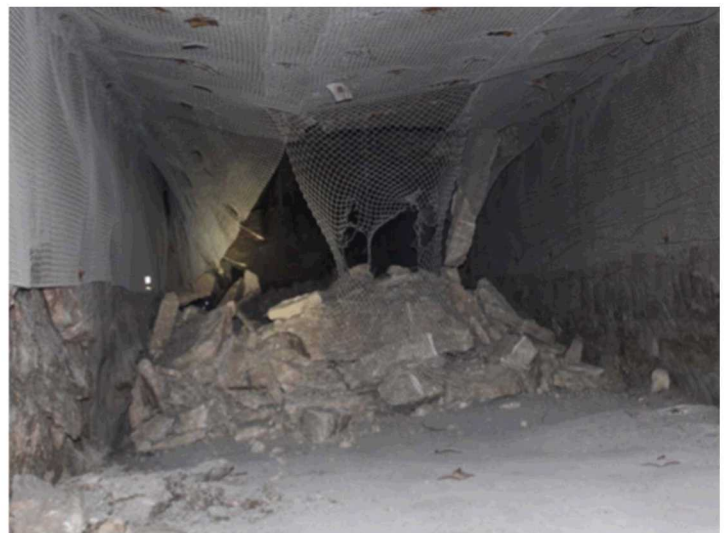
Figure 1. Roof collapse and resulting rubble pile in ES300-S3650 access drift at WIPP (from Carrasco 2019).
