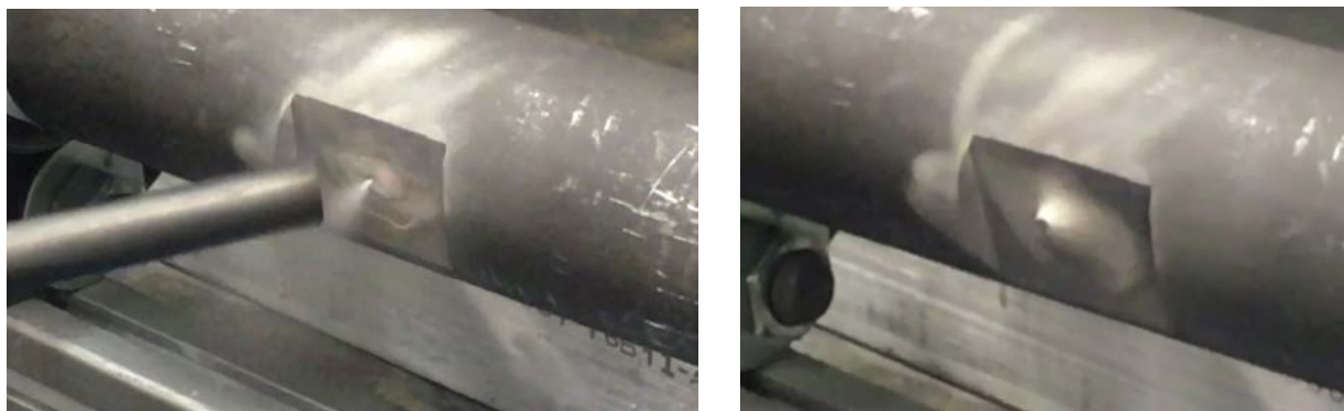
Figure 12. Repair of active leak using cold spray by VRC Metal Systems. Left: water leak; right: final repair. Pressure of the pipe was 1,000 PSI during and after the repair.
