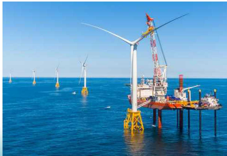
GE-Haliade 6 MW Turbines 30 MW Block Island Wind Farm Rhode Island
