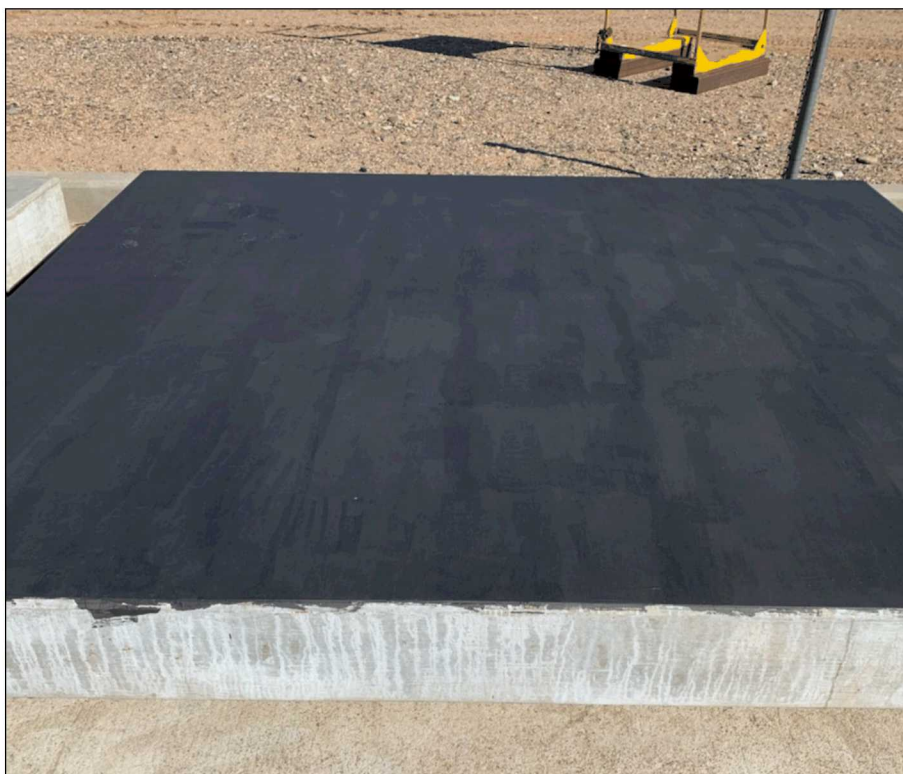
Figure 26. Dark base concrete wall coating application
