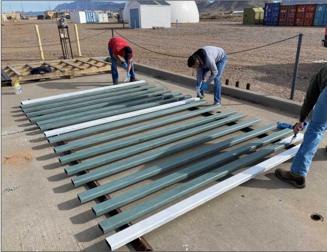
Figure 23. Light-base steel beam coating application
