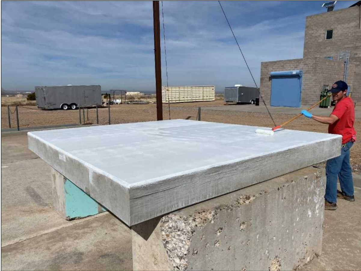
Figure 5. Application of light base coating on concrete wall
