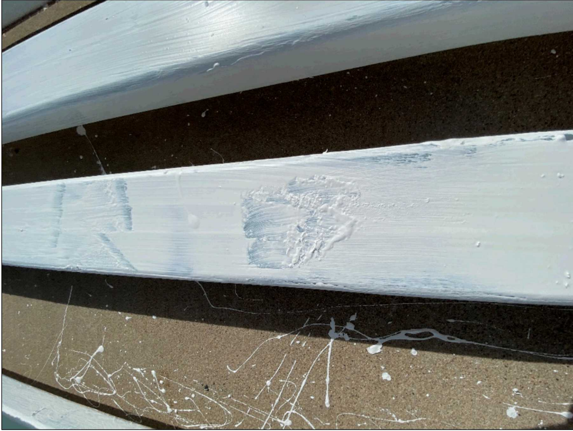
Figure 4. Light-base application issues on DOS steel picket fence
