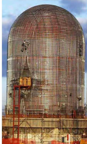
Figure 6. Tendons bending around an equipment hatch penetration in a 1:4-scale PCCV. [7]
