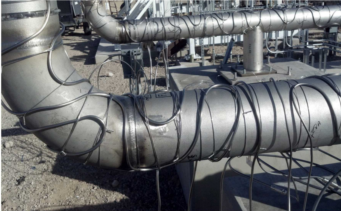
Figure 6: MI Cable Piping Serpentine Installation Attachment Wires
