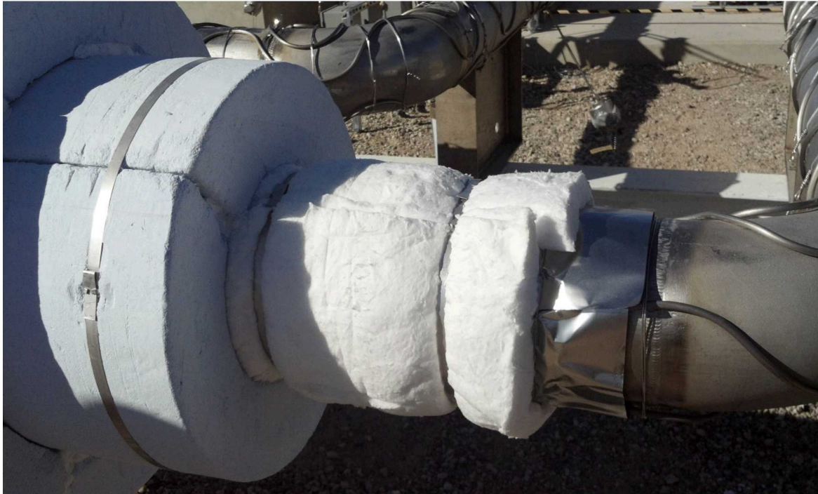
Figure 7: MI Cable Attachment Followed by Foil, Ceramic Blanket, 2 Layers of Perlite
