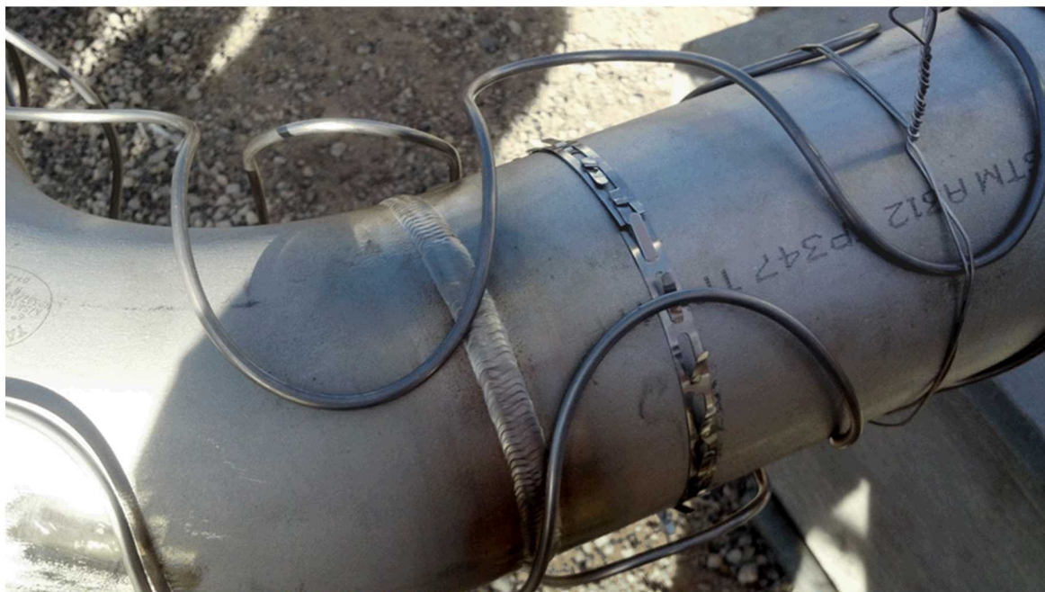
Figure 7: MI Cable Serpentine Pattern Formed onto Pipe
