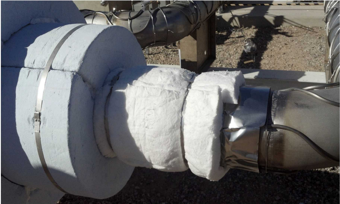
Figure 9: MI Cable Attachment Followed by Foil, Ceramic Blanket, 2 Layers of Perlite
