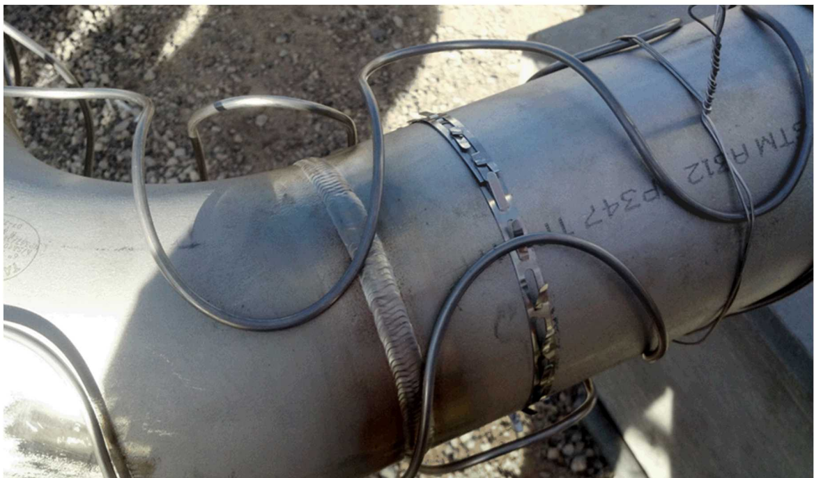
Figure 7: MI Cable Serpentine Pattern Formed onto Pipe
