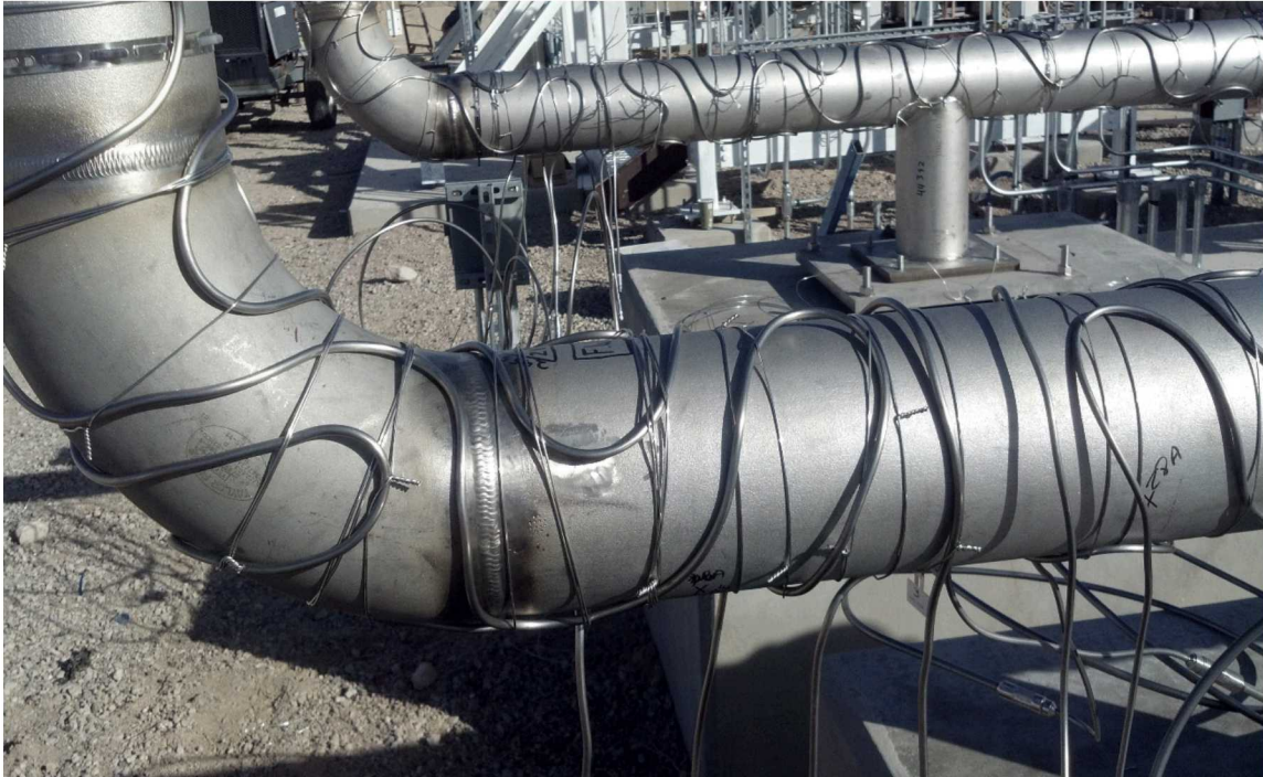
Figure 8: MI Cable Piping Serpentine Installation Attachment Wires
