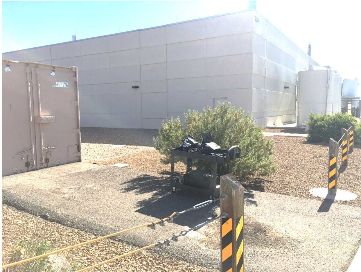
Figure 23: Monitoring location on the east side of building 720.
