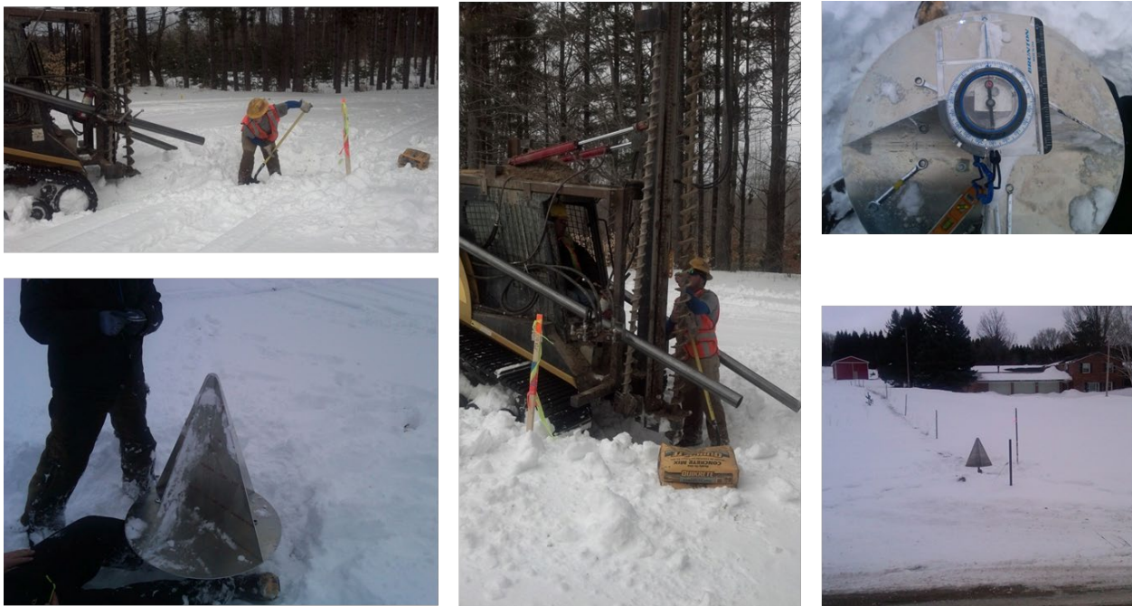
Figure 2-8. Photographs documenting the installation of the ACRs
