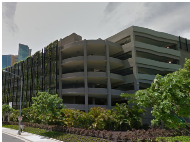
Ward Village Shops, Honolulu, HI. Image courtesy: Howard Hughes Corporation
