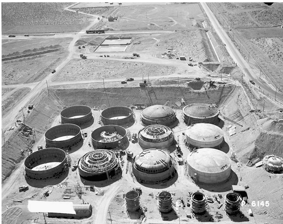
Fig. 1. An aerial view of the single-shell tanks (SST) under construction at Hanford site C-Farm, c. 1944. A total of 149 carbon steel SST with a design life of 20 years were built during 1943–1964. C-Farm was the first of the Hanford's SST farms selected for waste retrieval. Radioactive and chemical waste was pumped from C-Farm's twelve 100-series tanks (530,000 gal each), and four smaller 200-series tanks (55,000 gal each), and was sent to newer, double-shell tanks. At the time of this writing, the farm has been completely retrieved. The waste will be subsequently sent to the waste treatment and immobilization plan for the vitrification.
