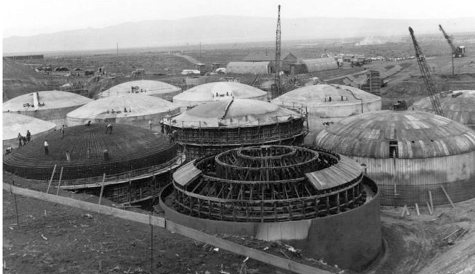
Fig. 2. An image of the double shell tanks under construction, c. 1970s. The construction of 28 double-shell tanks, with capacities up to 4400 m 3 and design lives of 50 years, began in 1968.
